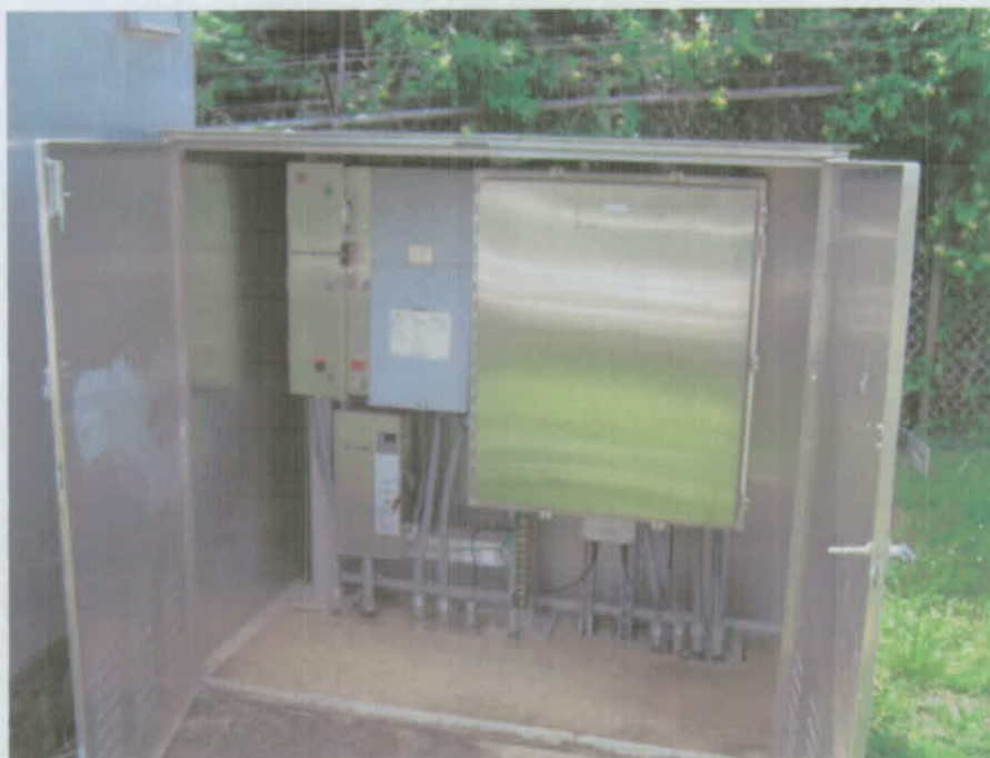
Photograph 4 – RW Control Enclosure
