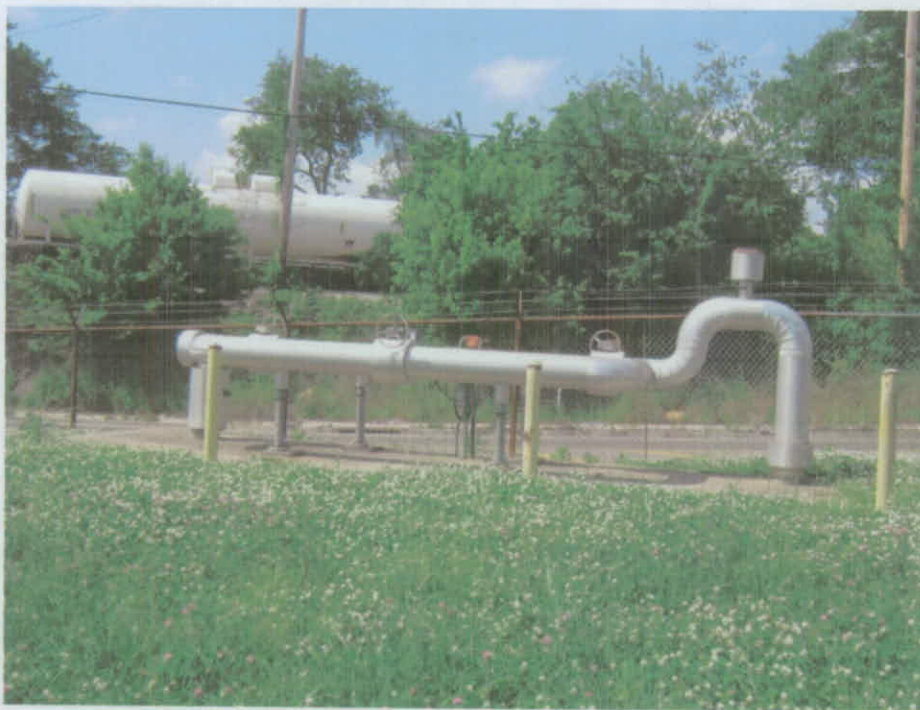
Photograph 6 – Sanitary Sewer Discharge Loop
