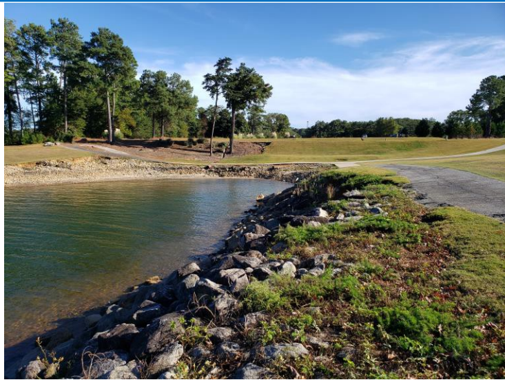
Photo 15: Armoring located on the side of Lake Lanier at the Project Site.
