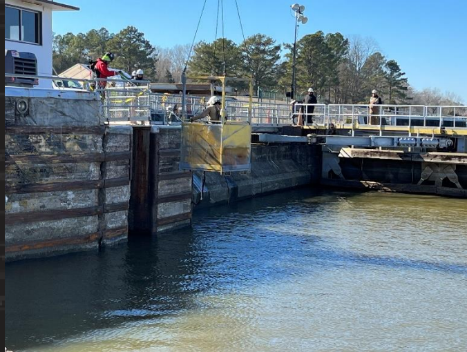
Diver Inspecting Stoplog Slot
