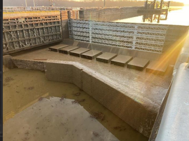
Damaged Sill
