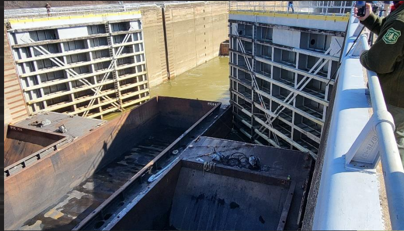
Lower Miter Gates Closing
