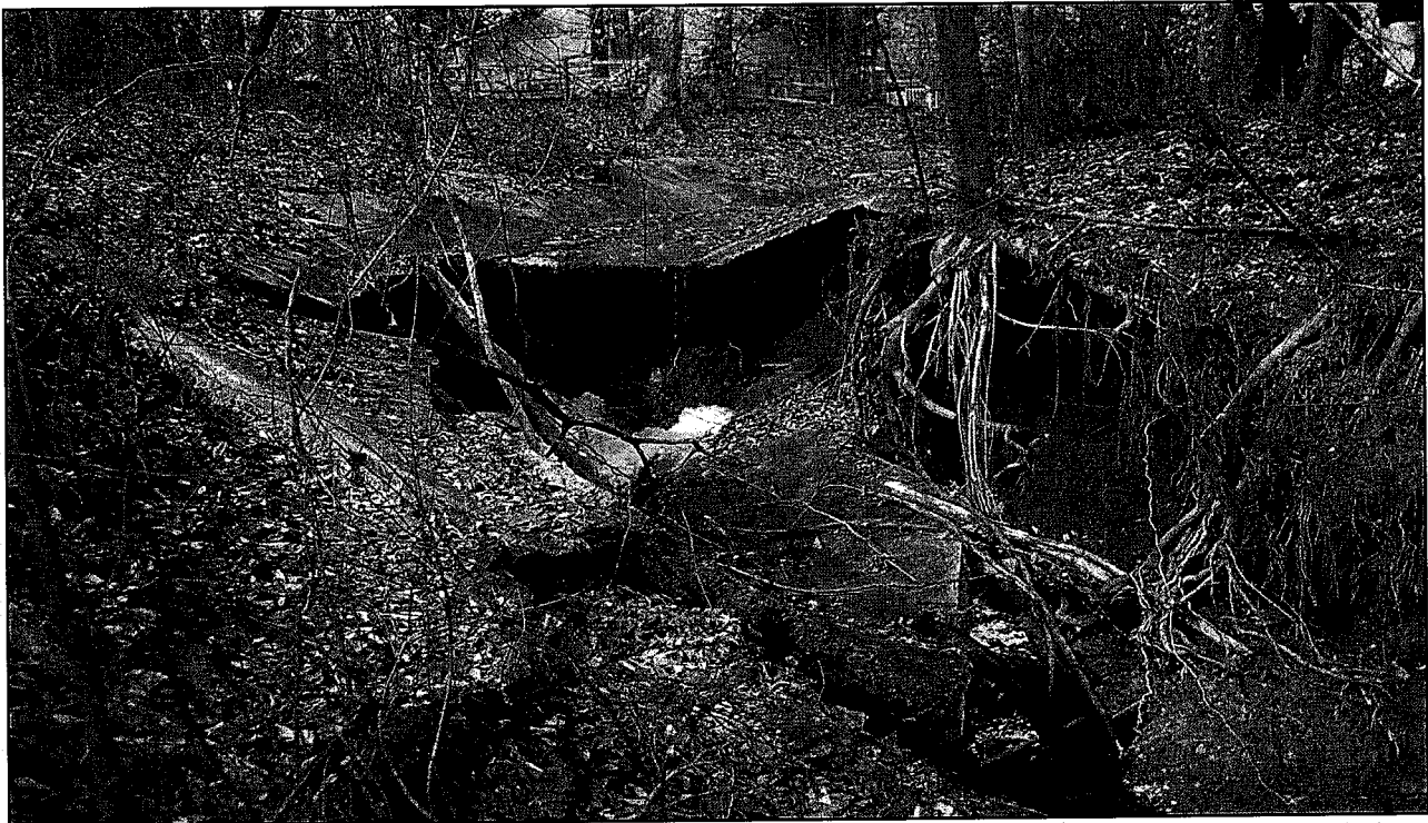
Figure 3: Shows the under cutting of the wet pond concrete spillway and the loss of about 25 feet of the spillway embankment putting the project in eminent danger of failure and is creating a safety hazard for the community children playing in the area.
