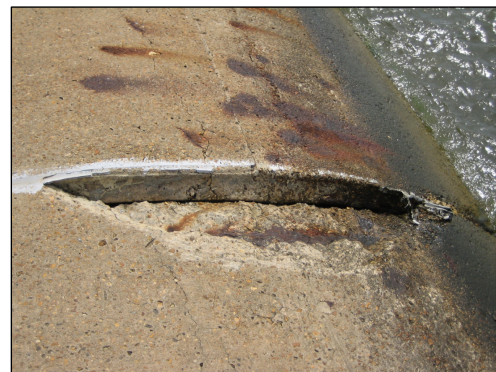
Figure 2.3.13-7. Damaged Seawall Joint with Exposed Reinforcing Steel
