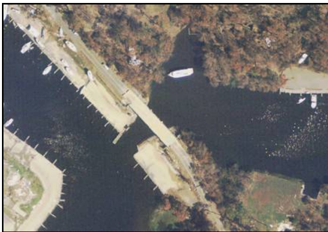
Figure 2.3.11-3. Aerial view of Shearwater Bridge
