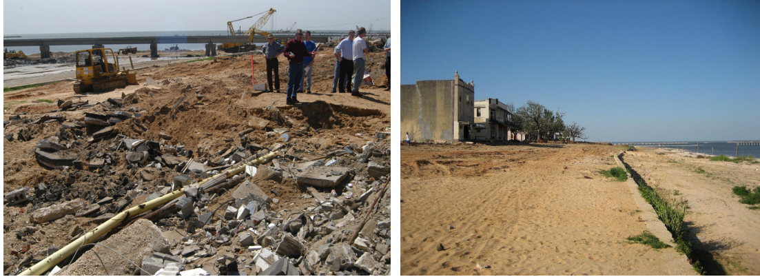
Figure 2.3.6-2. Downtown Bay St. Louis, After Hurricane Katrina
