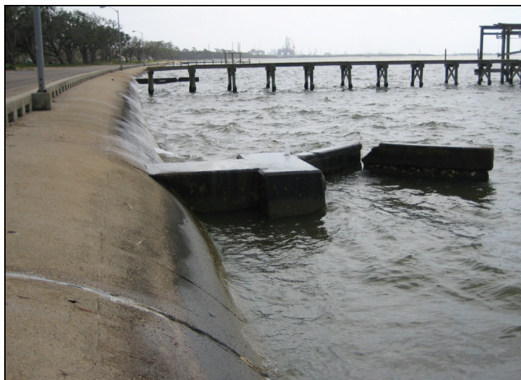
Figure 2.3.13-4. Concave Seawall, Culvert Outfall, and Pier, Looking East Beach Boulevard Is to the Left
