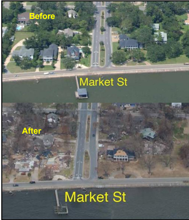
Figure 2.3.13-5. Pascagoula Beach Boulevard Before and After Hurricane Katrina
