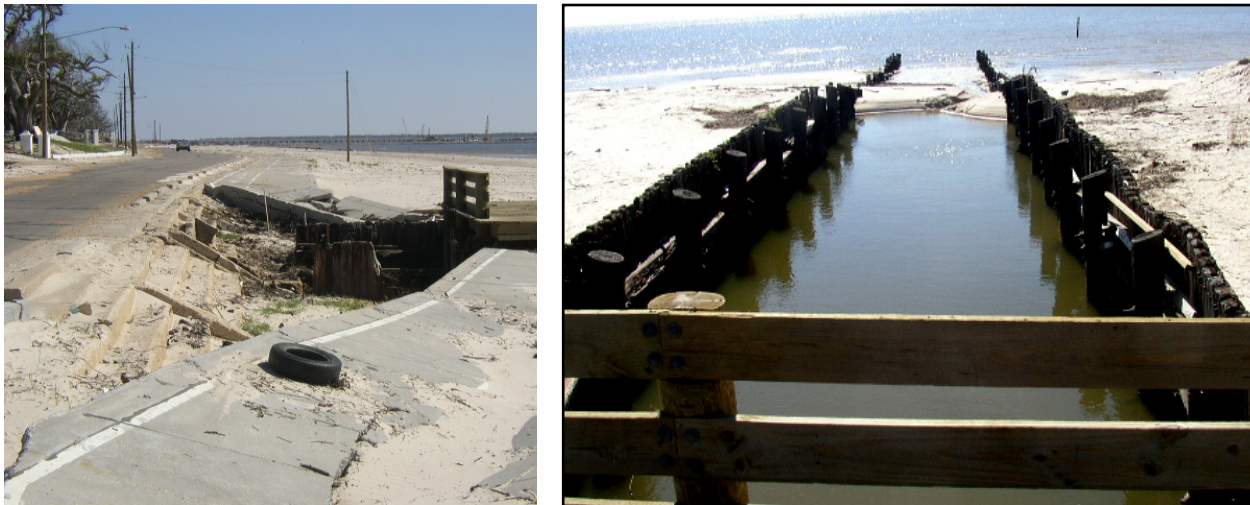
Figure 2.3.4-4. Damaged Pathway, Drainage Channel Outlet, and Outlet Bridge, Near Waveland
