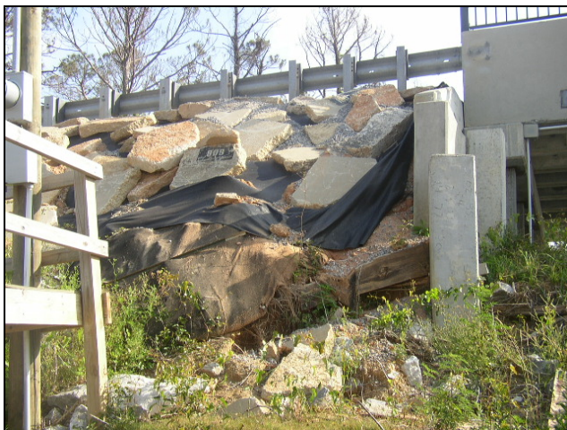
Figure 2.3.11-4. Timber Wall Failure at North Abutment
