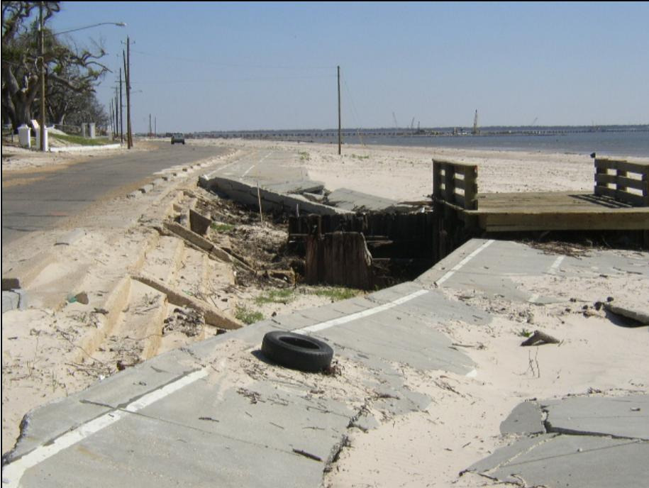
**Figure 4. Damaged Pathway, Drainage Channel Outlet, and Outlet Bridge, Near Waveland. Beach Road and Seawall Beyond.**
