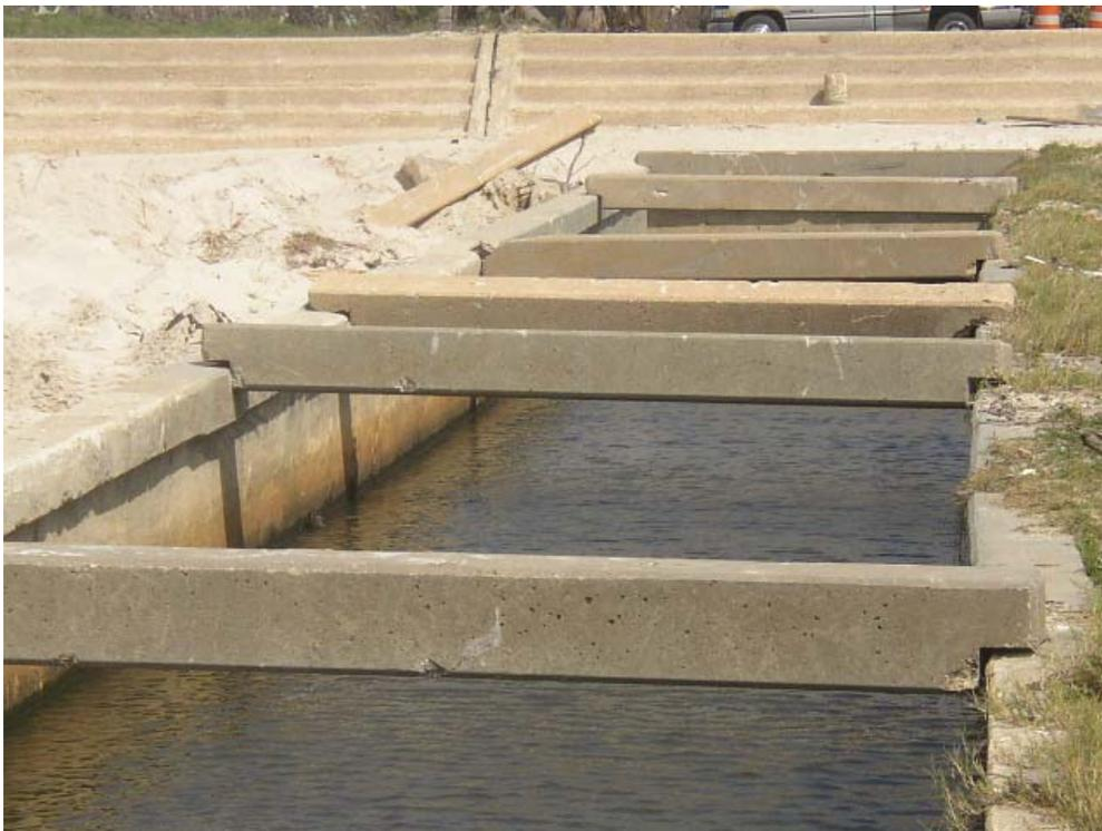
**Figure 6. Drainage channel, looking towards the seawall. Broken braces are shown stacked on the beach to the left of the channel. 3 April 2006 photo**
