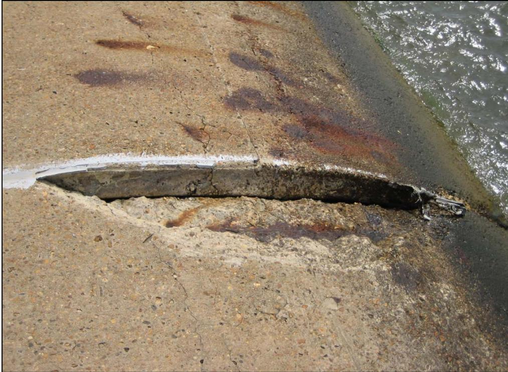
**Figure 11. Damaged Seawall Joint with Exposed Reinforcement Steel.**
