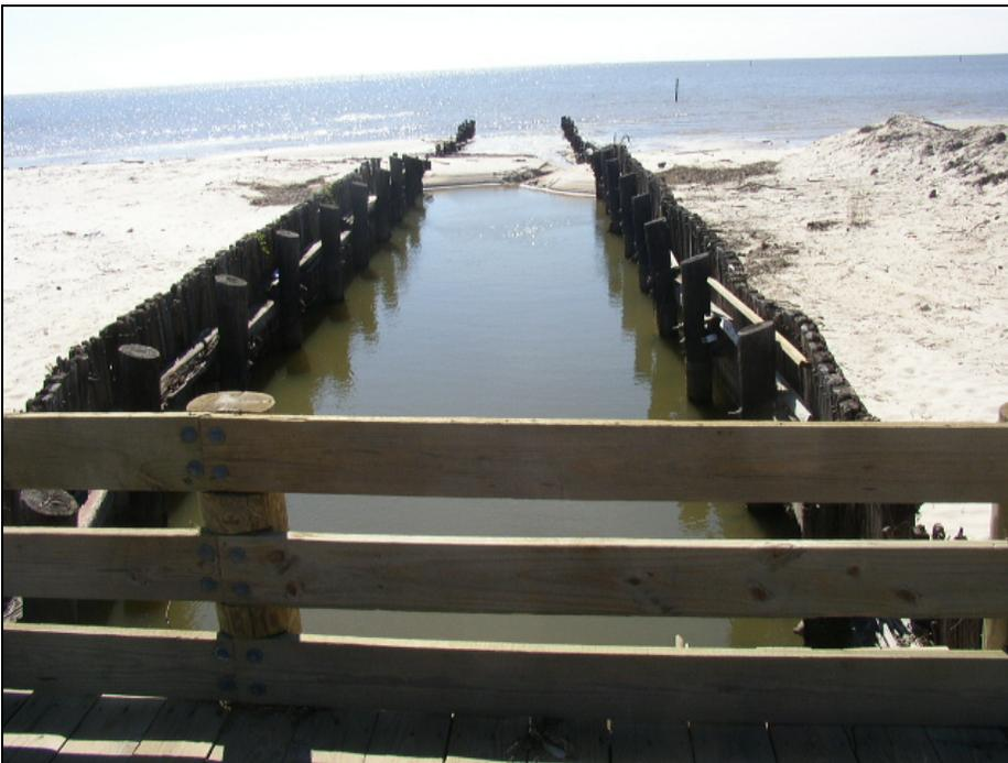
**Figure 5. Channel Outlet. Outlet is Breached, Extension Walls are Damaged, and Outlet is Choked with Sand.**
