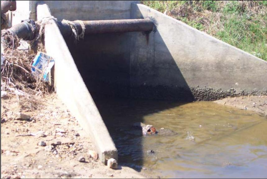
**Figure 7. Landward entrance of outlet channel drainage culvert.**
