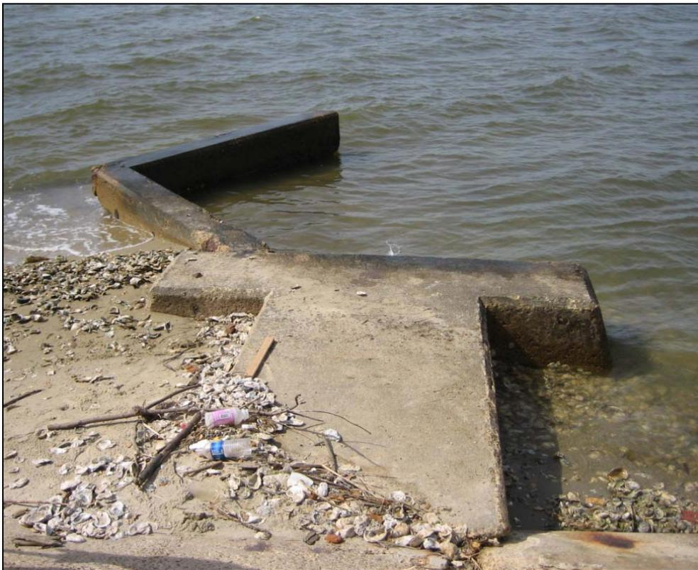
**Figure 6. Concrete Culvert Outfall Monolith and Chevron Deflector, Near Spanish Point.**
