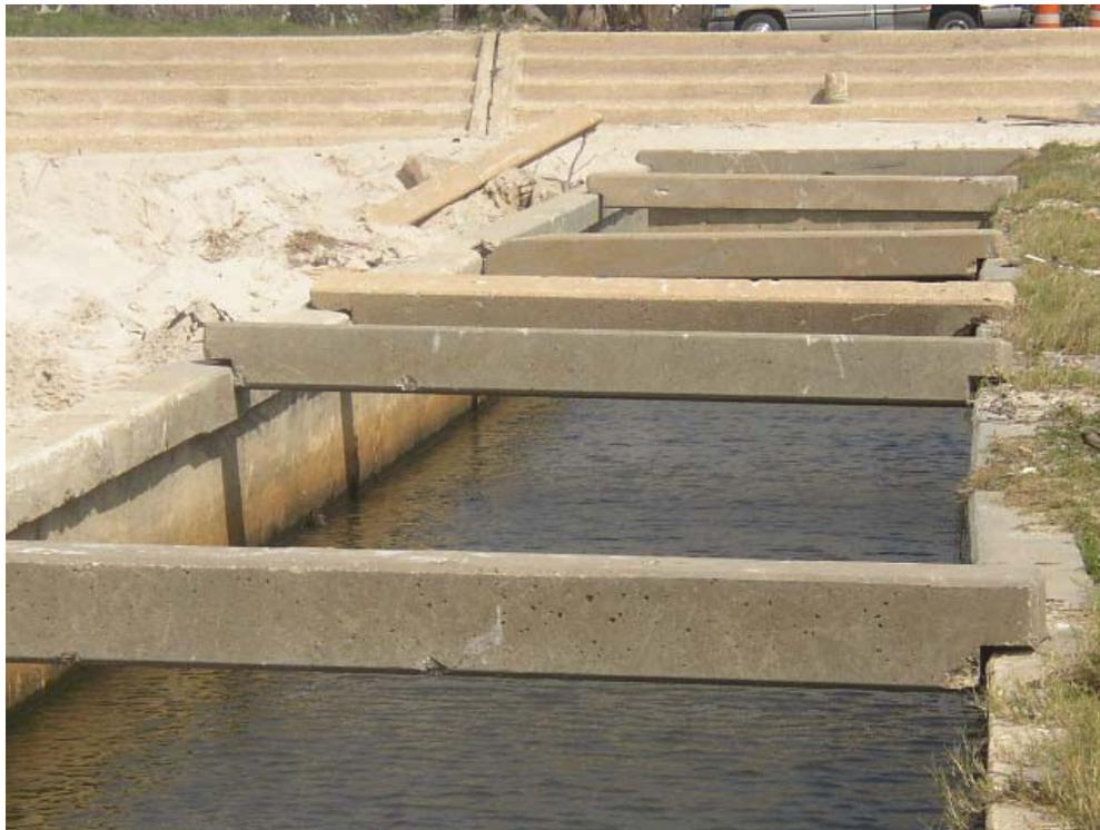
**Figure 7. Drainage channel, looking towards the beach. Ends of braces are cracked or broken, and all braces show impact damage on at least one surface 3 April 2006 photo.**
