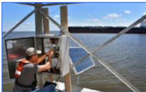
Sitting atop the U.S. Coast Guard navigation range in Mobile Bay, Mobile District coastal engineer, Richard Allen, connects newly installed gauges that measure water level, wave height, turbidity, salinity and suspended-sediment concentration.
