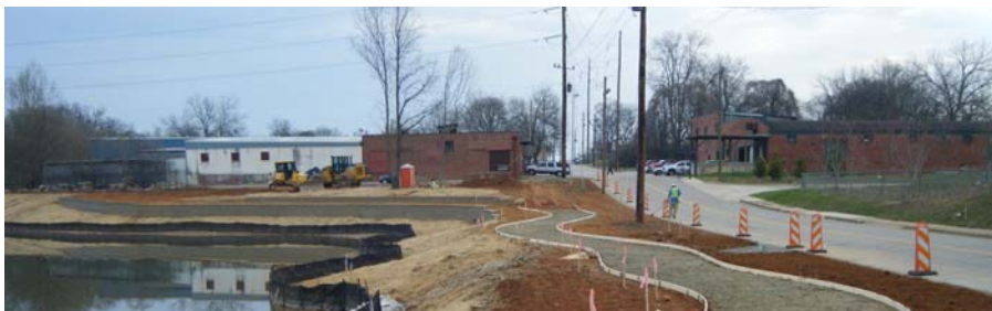
Regional stormwater detention facility adjacent to stream restoration partially funded by a 319(h) grant in the headwaters part of Flat Creek.
