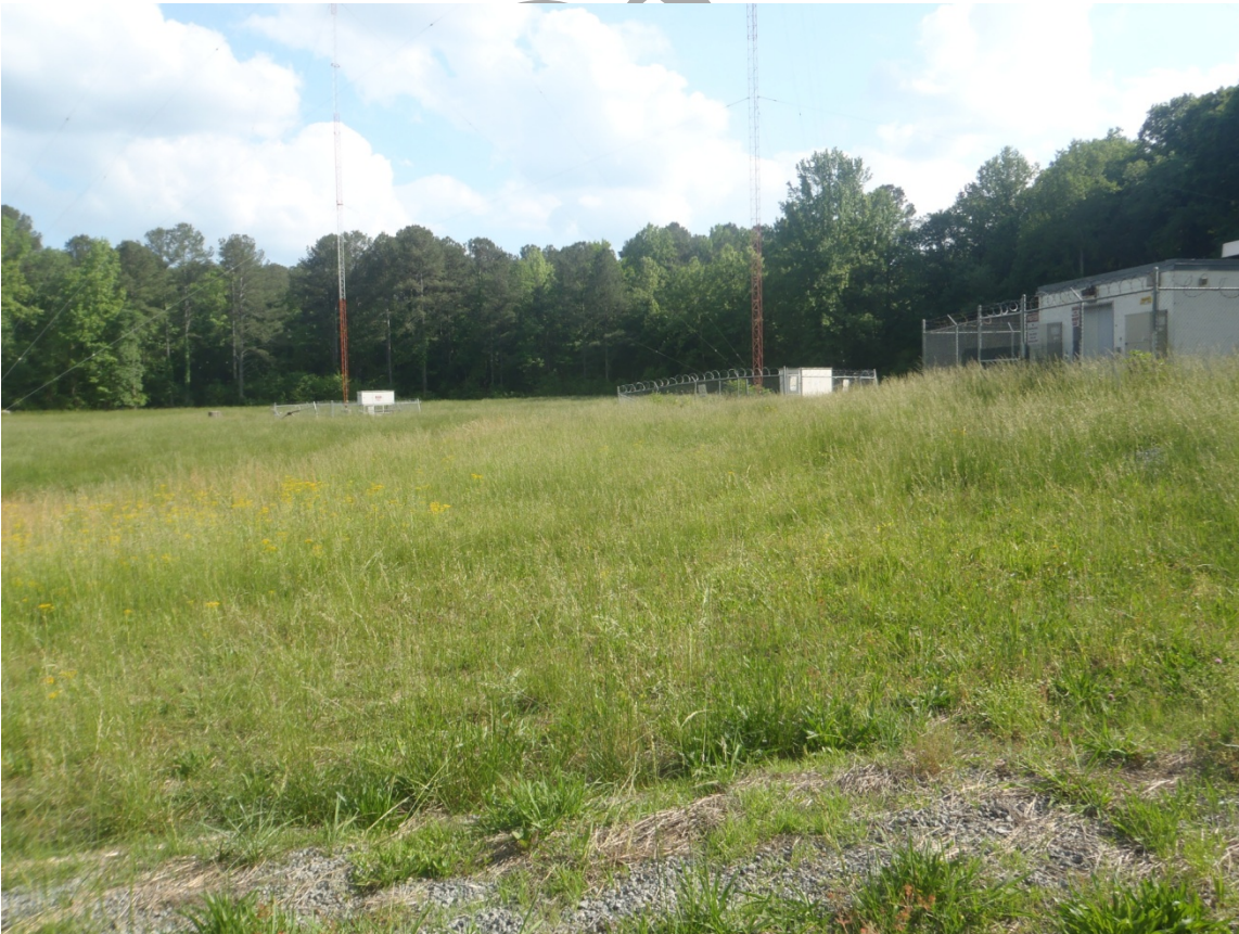
Photograph 24 - Two radio towers and associated structure adjacent to Alternative B70
