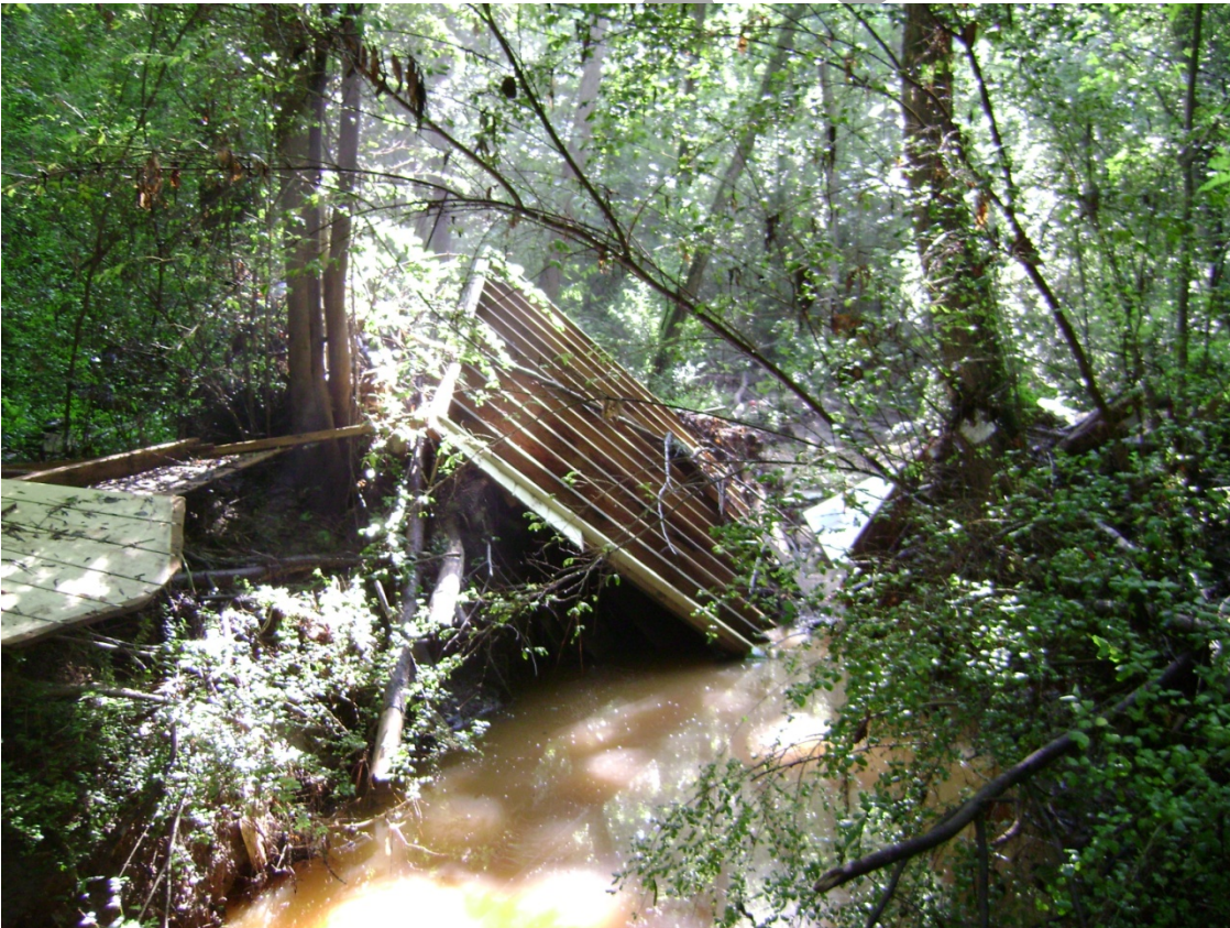
Photograph 18 - Destroyed shed found at Alternative B2-1
