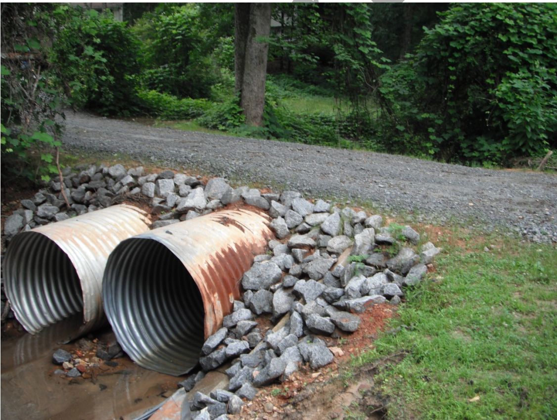
Photograph 20 - Gravel drive and culvert at Alternative B3-2-3
