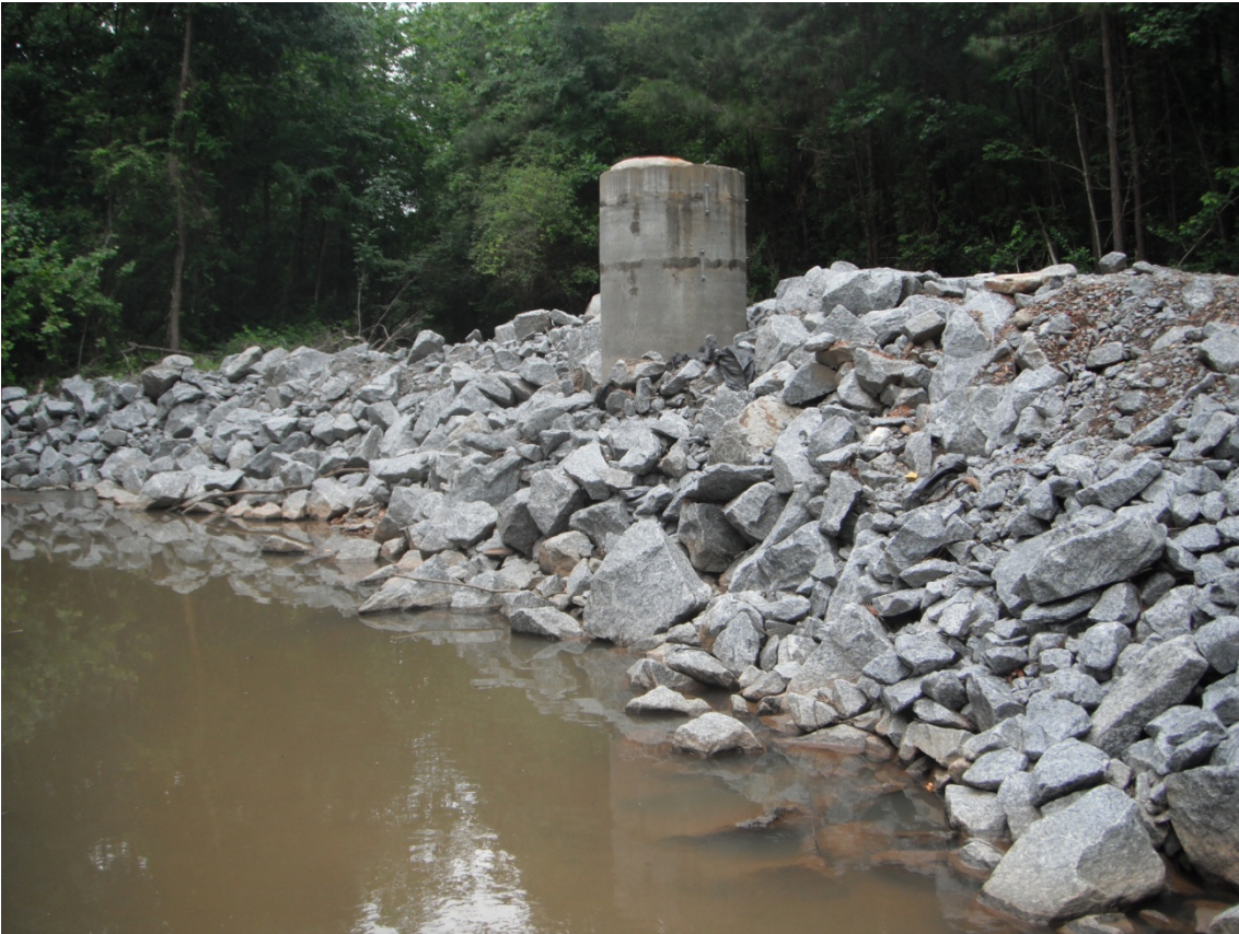
Photograph 21 - Rip-rap wall with sewer manhole at Alternative B4-1
