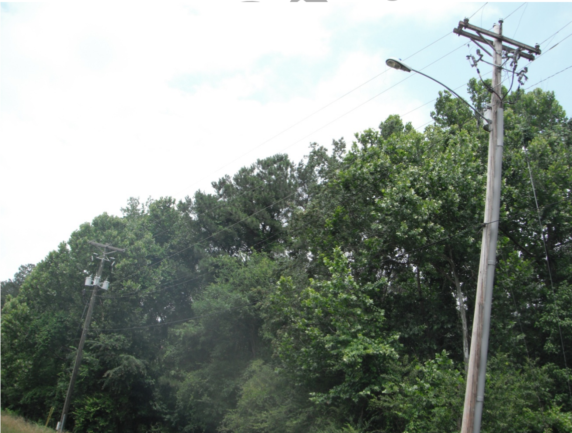
Photograph 26 - Transformers observed at Alternative B70
