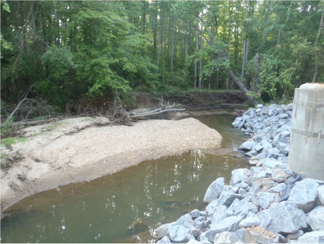
Photograph 5 - Alternative B4-1 looking downstream with rip-rap wall on the right bank
