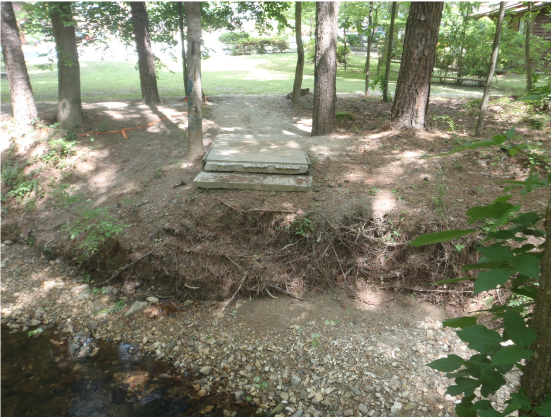
Photograph 19 - Collapsed footbridge at Alternative B3-2
