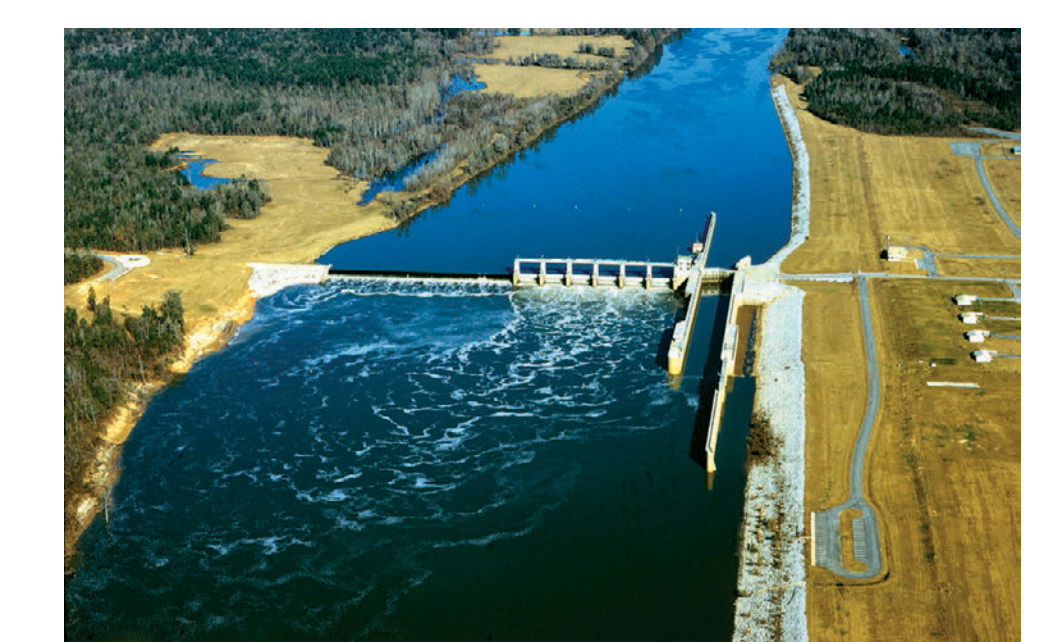
Claiborne Lock and Dam
