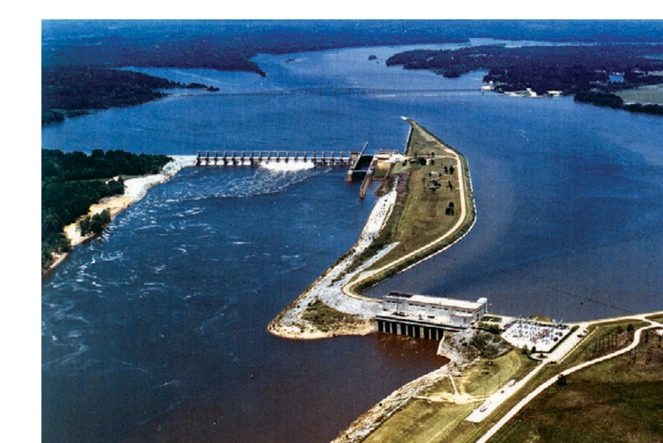
Millers Ferry Lock and Dam
