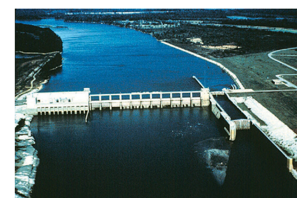
R.F. Henry Lock and Dam
