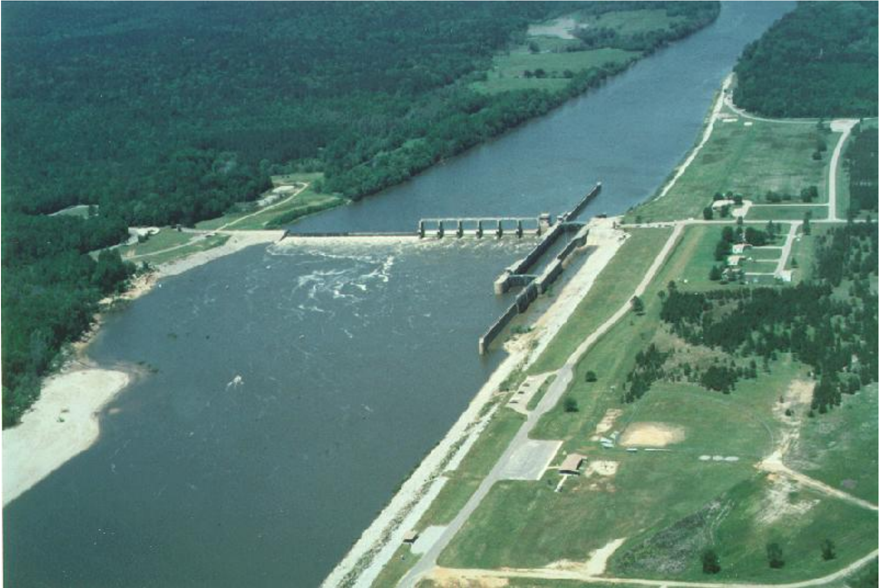
Figure K.30 Photo of Claiborne Lock and Dam
