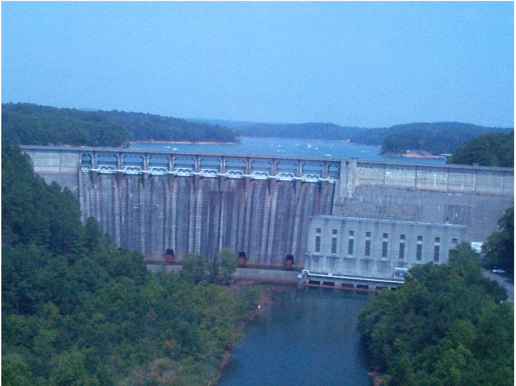
Figure B.02 Photo of Allatoona Dam
