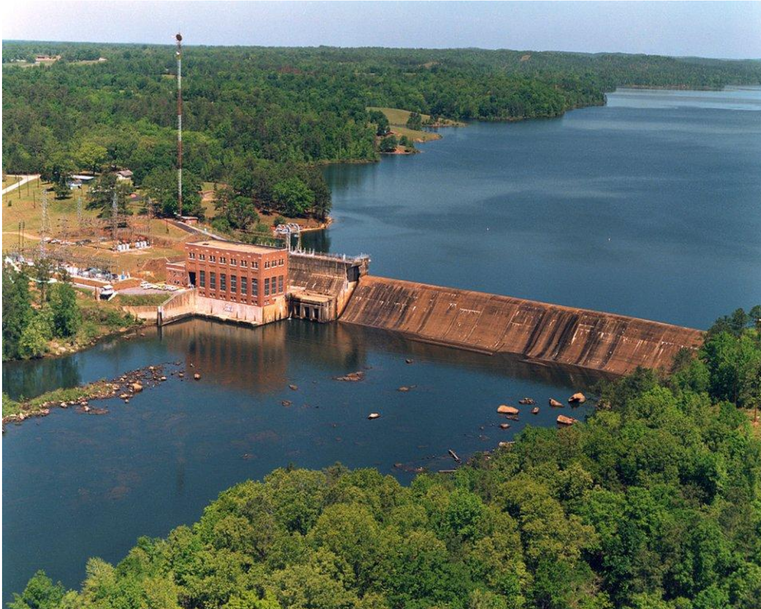
Figure K.16 Photo of Yates Dam
