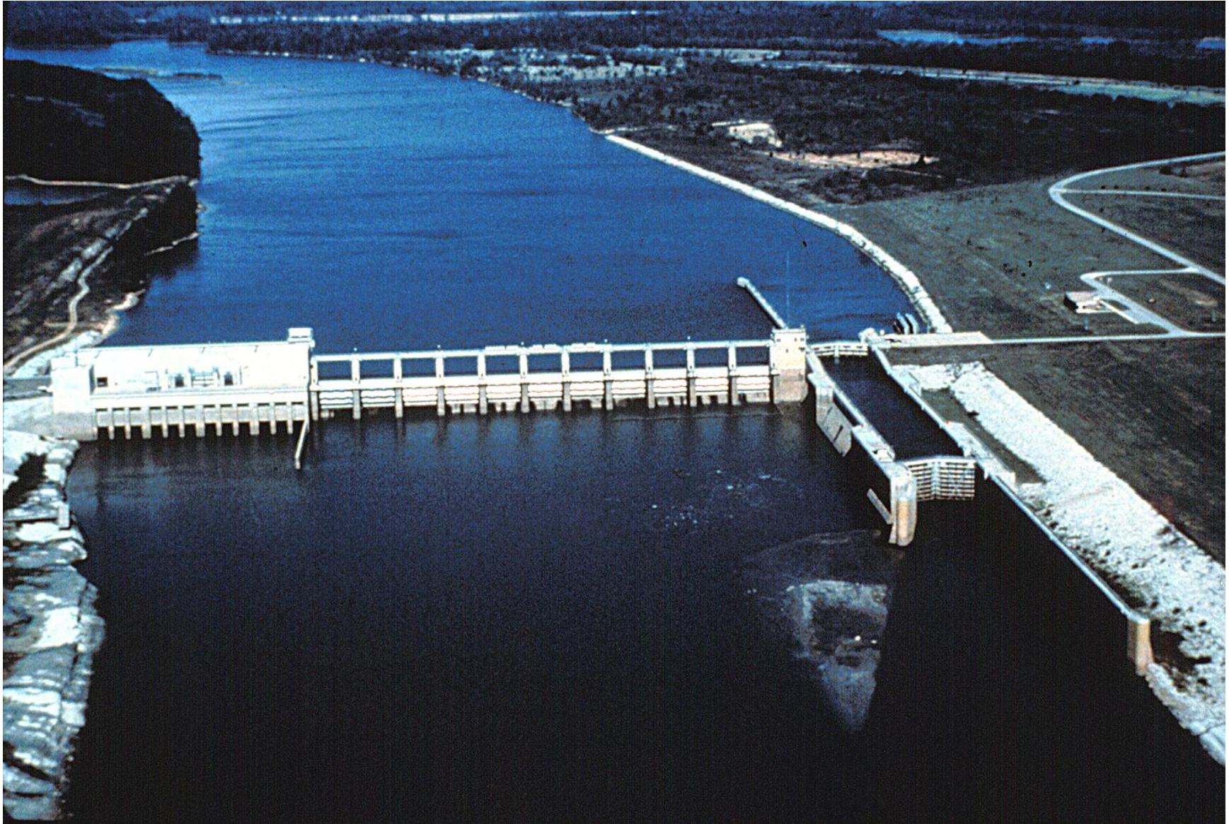
Figure C.02 Photo of Robert F. Henry Lock and Dam
