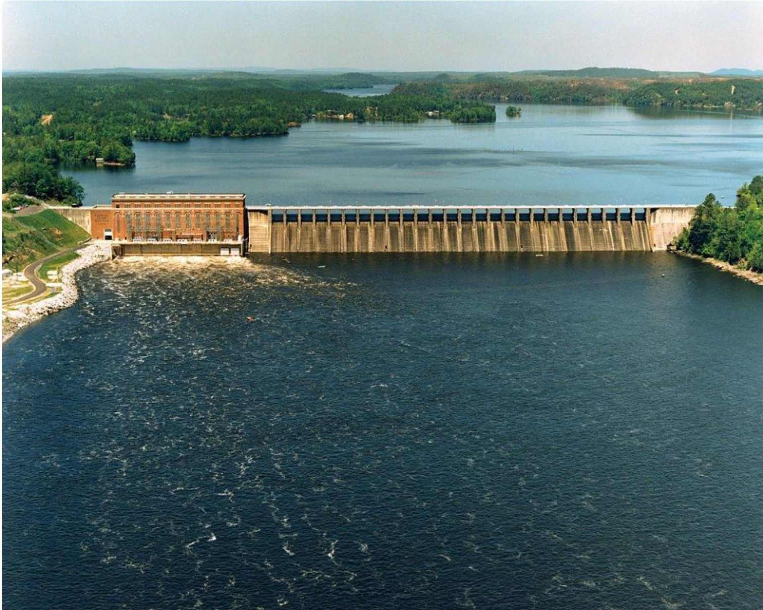
Figure K.02 Photo of Lay Dam
