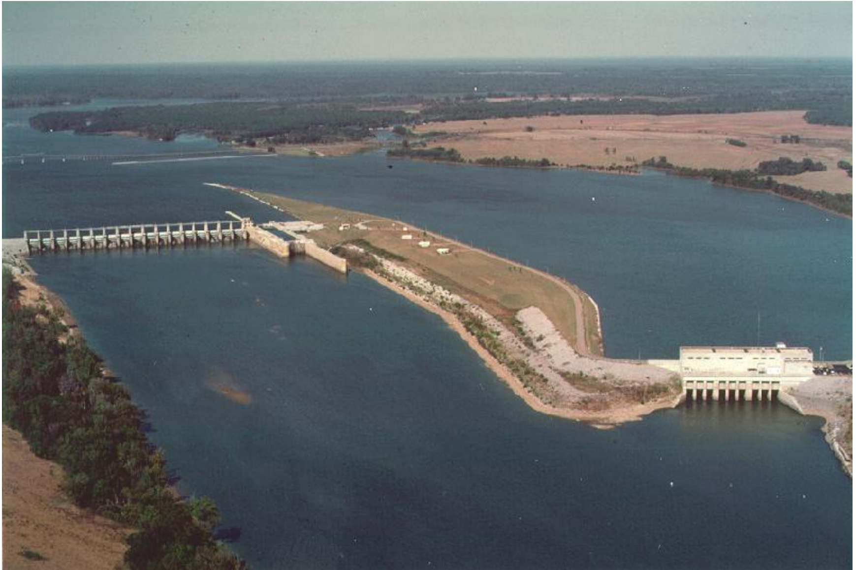
Figure D.02 Photo of Millers Ferry Lock and Dam
