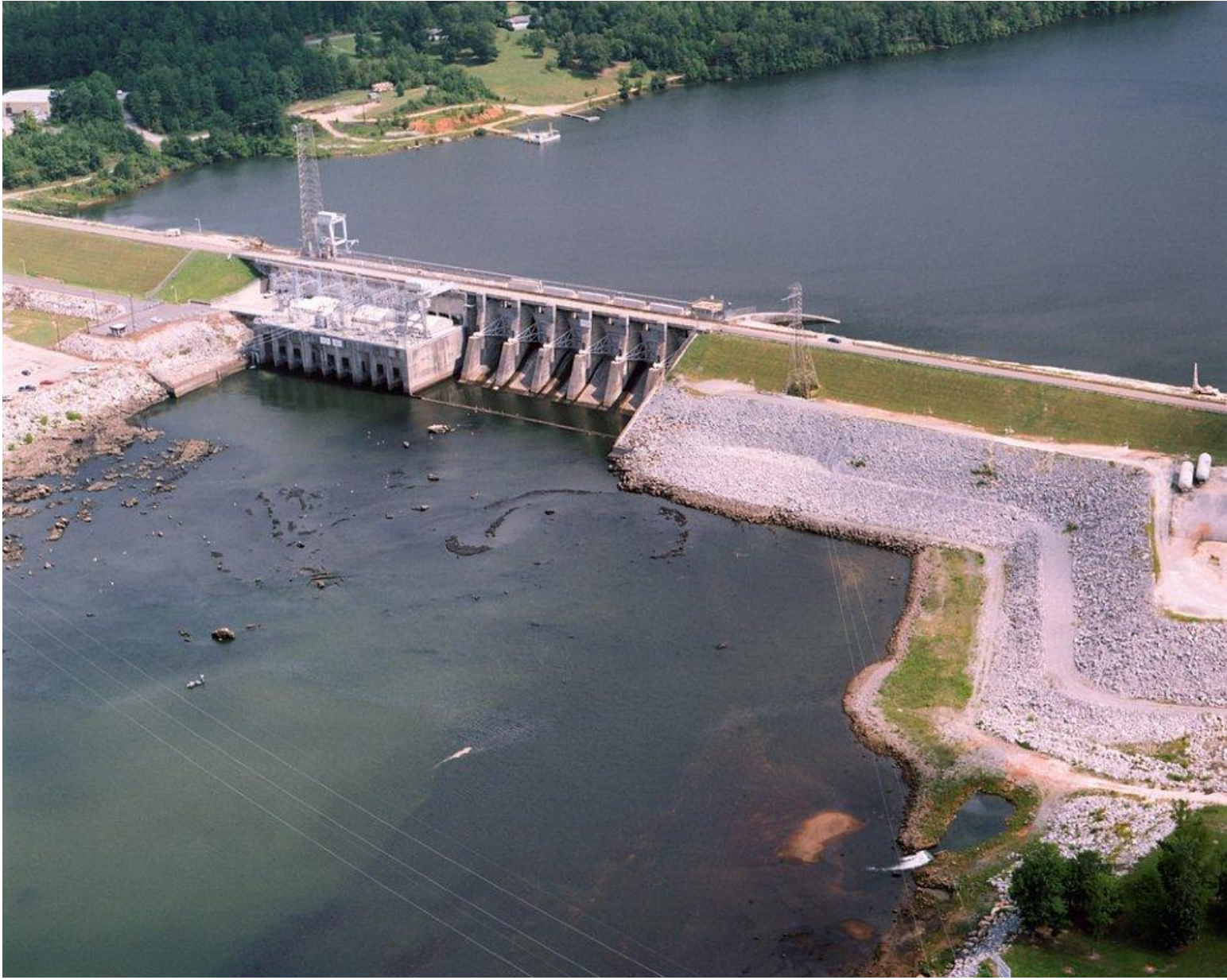
Figure G.02 Photo of Logan Martin Dam
