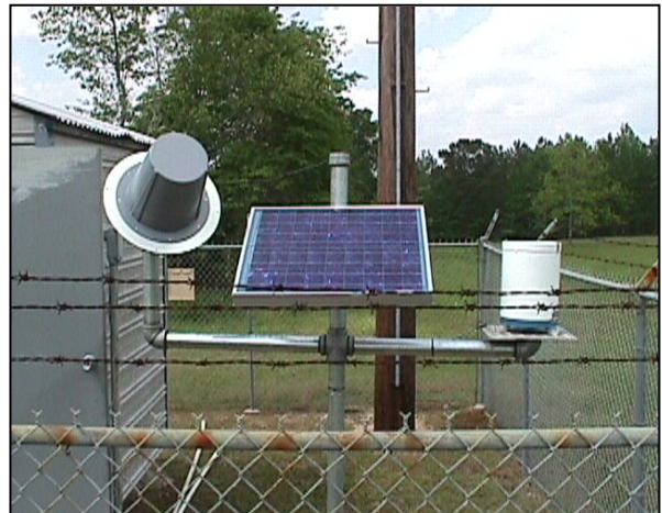
Figure 5-2. Typical field installation of a precipitation gage
