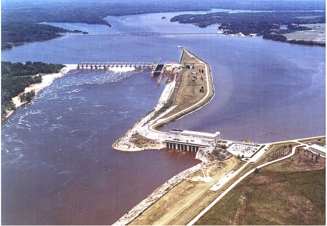
Millers Ferry Lock and Dam Alabama River, Alabama
