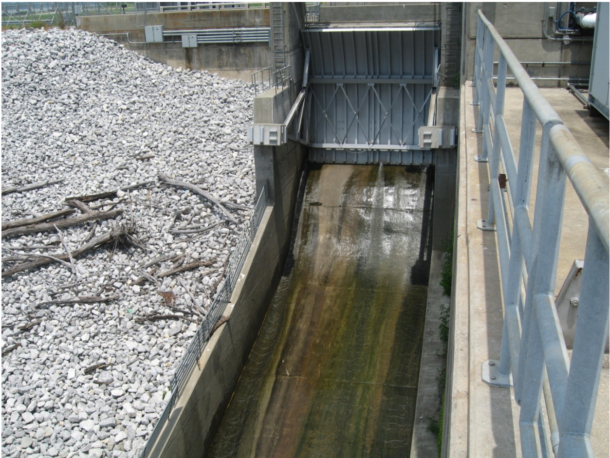
Figure 3-1. Trash Gate at Millers Ferry Project
