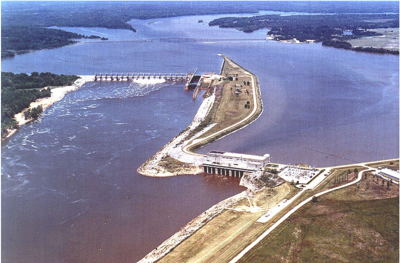
Figure 2-1. Millers Ferry Lock and Dam
