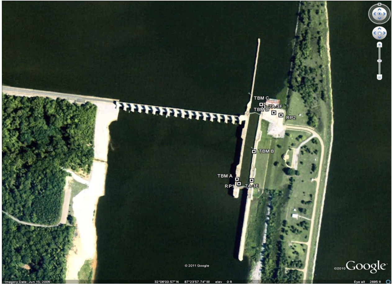
MILLERS FERRY LOCK AND DAM
