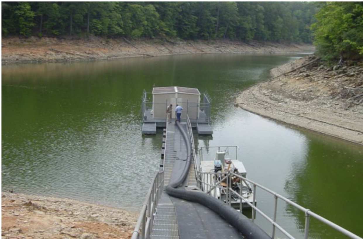
26 27 Figure 8-1. The city of Chatsworth Water Intake Structure
