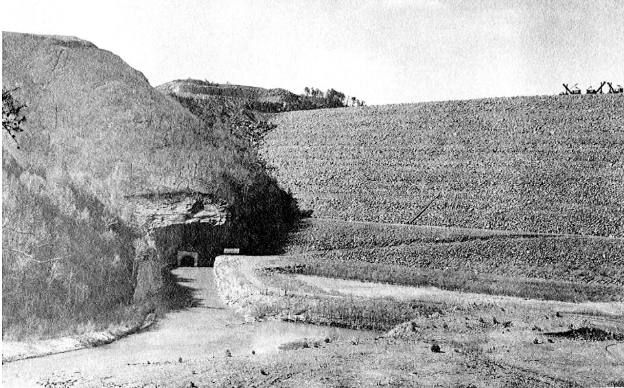
1 Figure 2-15. Diversion Tunnel Upstream Entrance Prior to Filling
