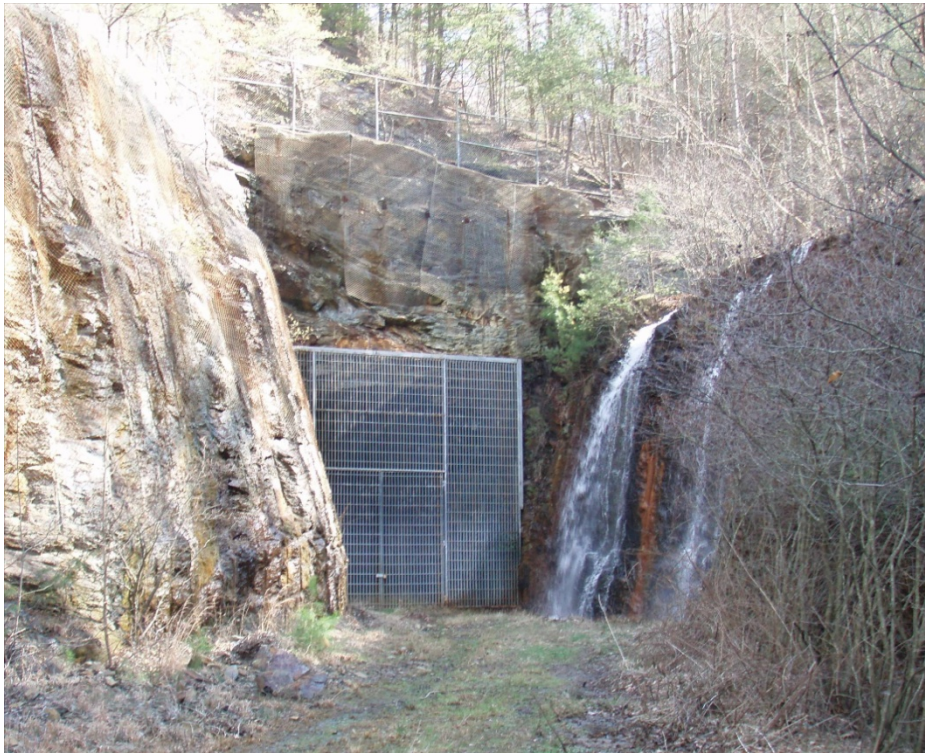
Figure 2-13. Downstream Opening of the Emergency Sluice Tunnel
