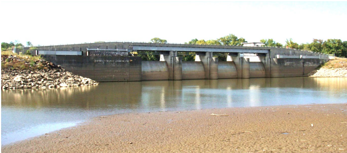
10 Figure 2–16. Reregulation Dam, Looking Downstream
