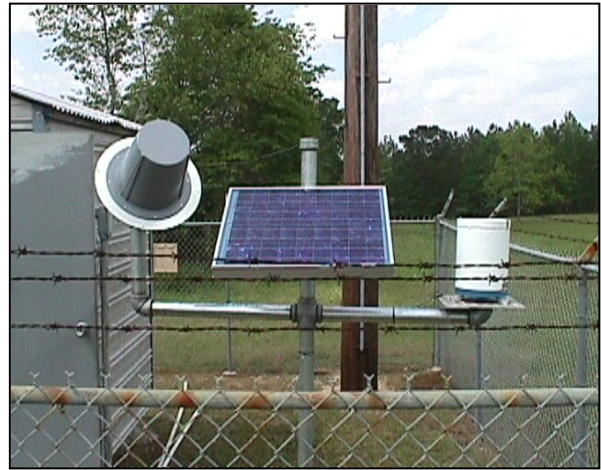
Figure 5-2. Typical field installation of a precipitation gage
