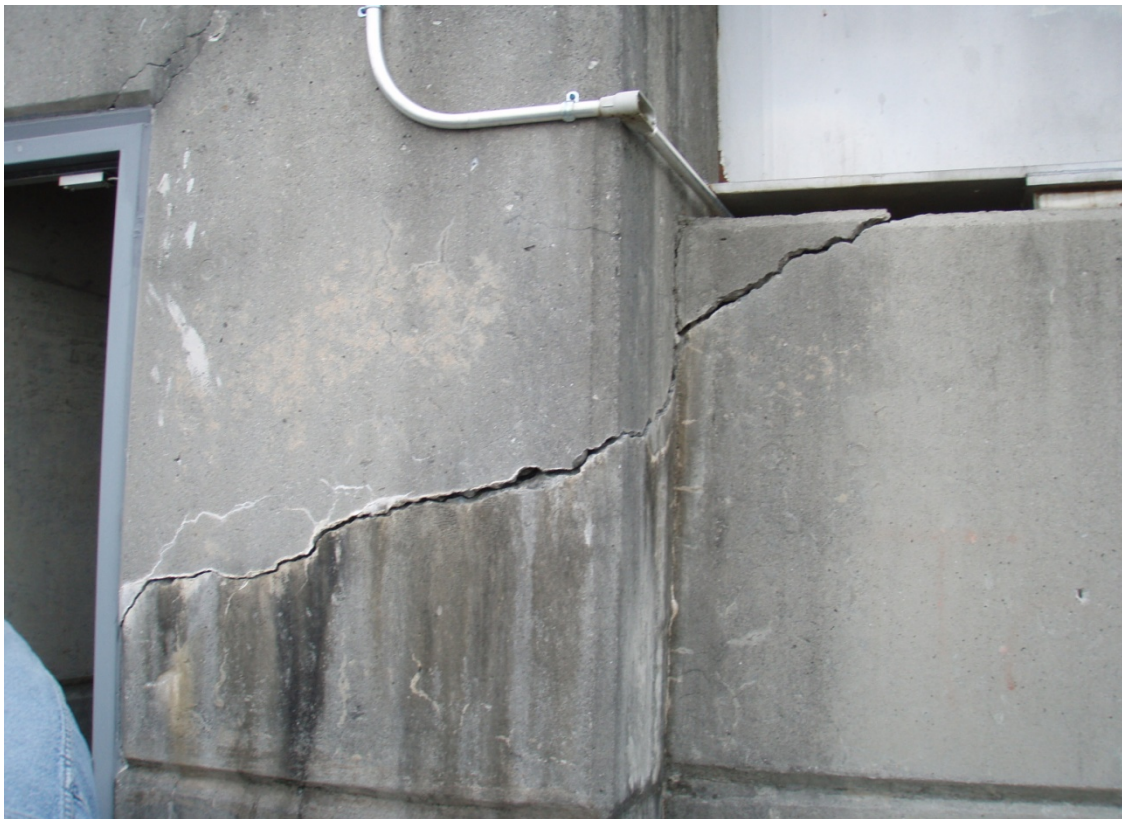
Figure 3-5. Close-up of crack on upstream side (east bridge end) of gate No. 4
