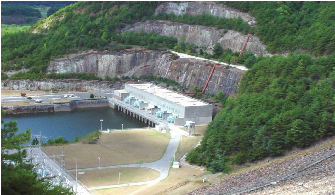
42 Figure 2-11. Carters Powerhouse at Tailrace
