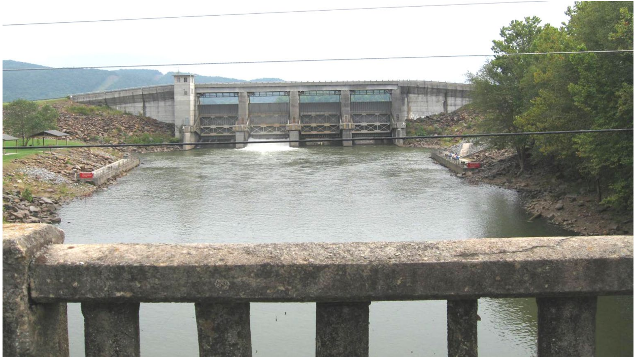
Figure 2-17. Reregulation Dam, Looking Upstream From Old US Hwy 411
