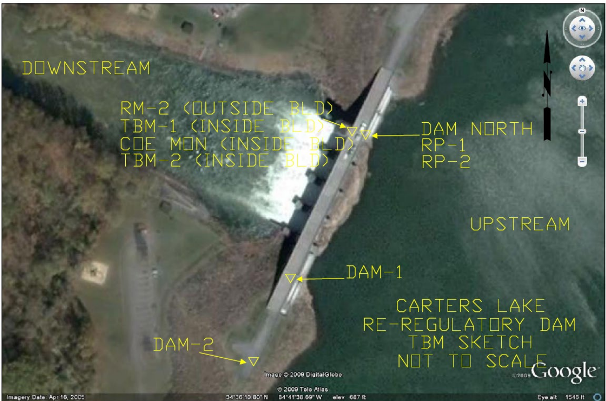
Carters Lake Reregulatory Dam
