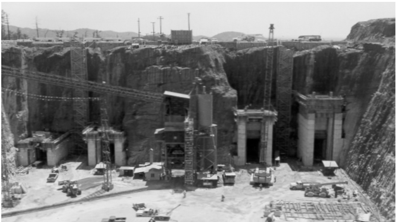
4 Figure 2-8. Upstream of Intake During Construction
