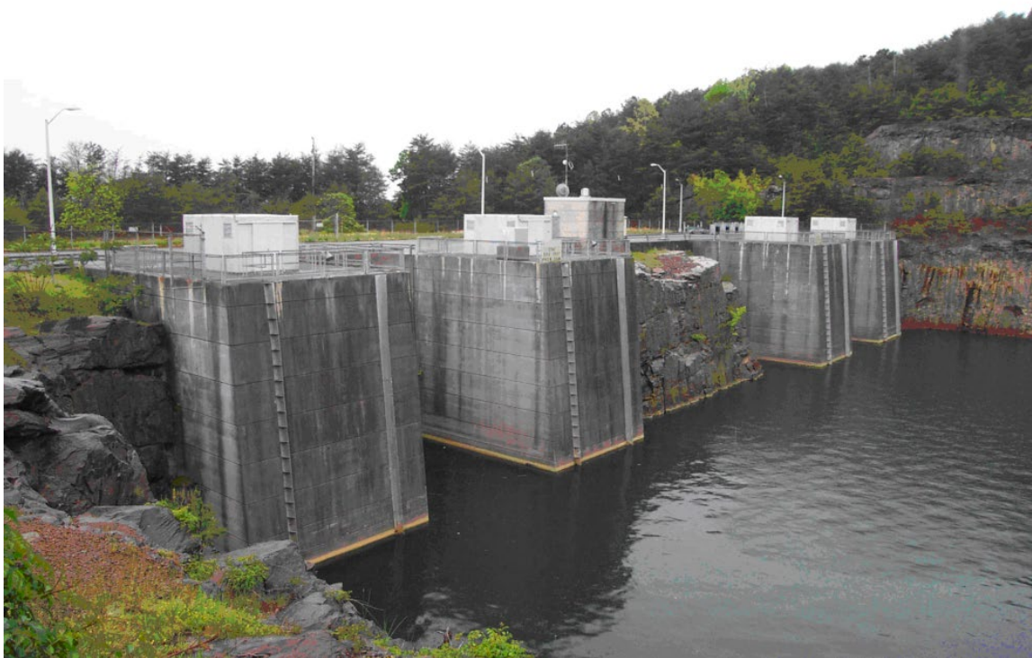
Figure 2-10. Intake Structure Looking Downstream
