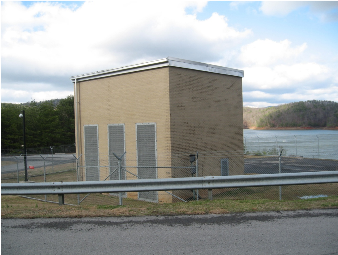
Figure 2-14. Low Level Sluice Control Building
