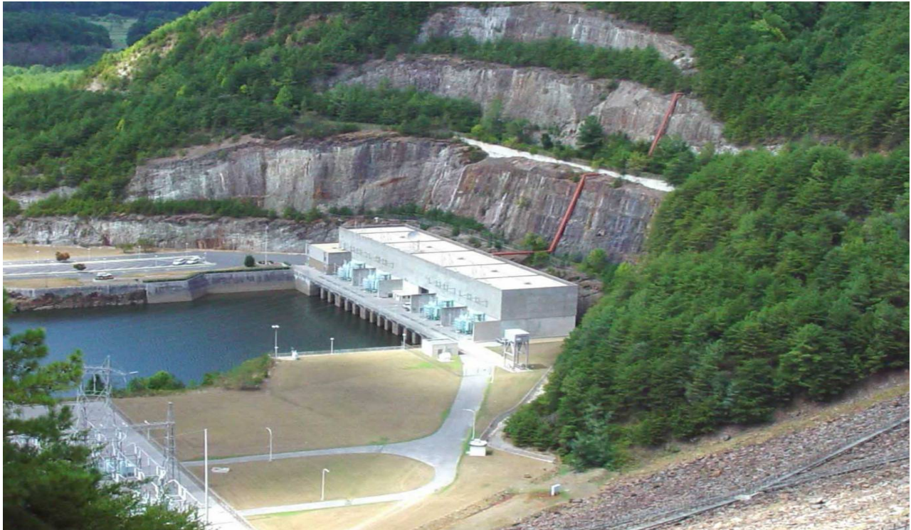
Figure 2-11. Carters Powerhouse at Tailrace
