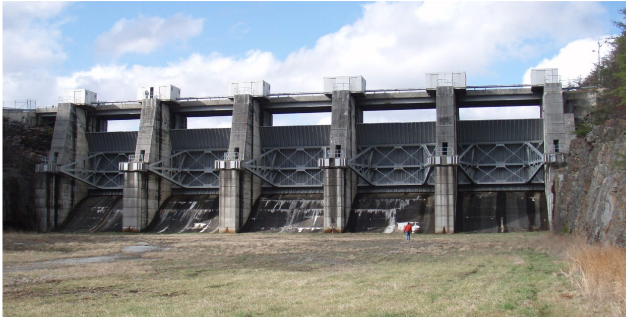
Figure 2-6. Emergency Gated Spillway (Looking Upstream)
