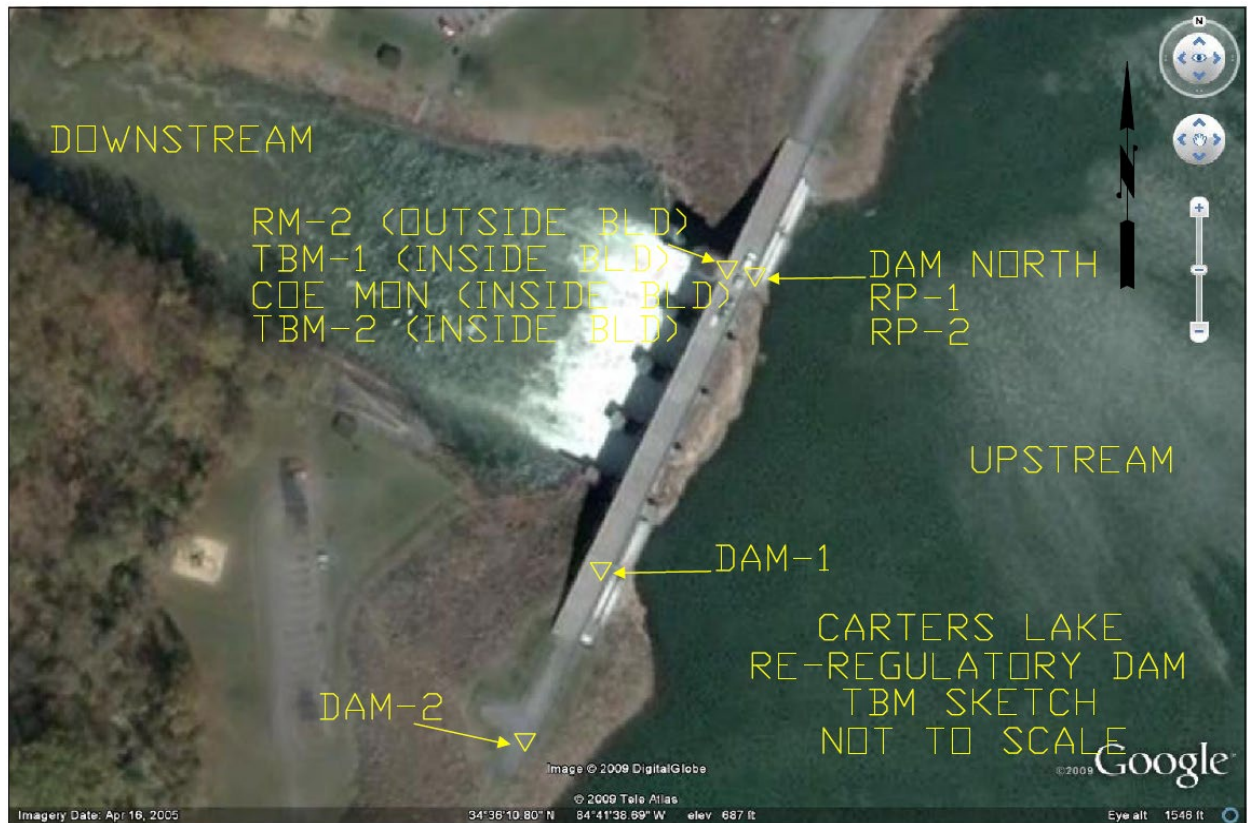
Carters Lake Reregulatory Dam
