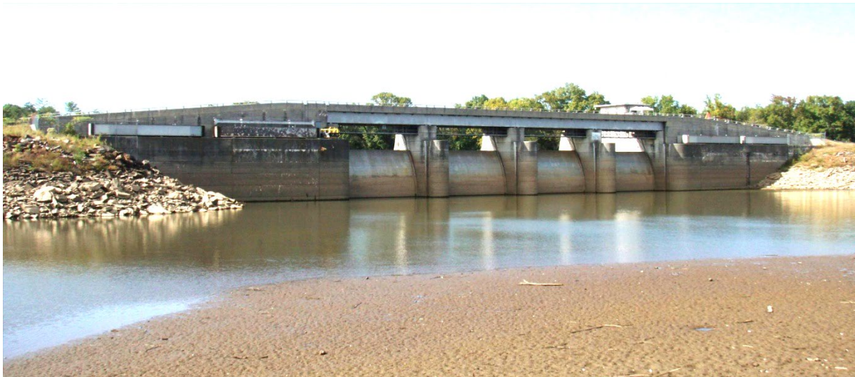
Figure 2-16. Reregulation Dam, Looking Downstream
