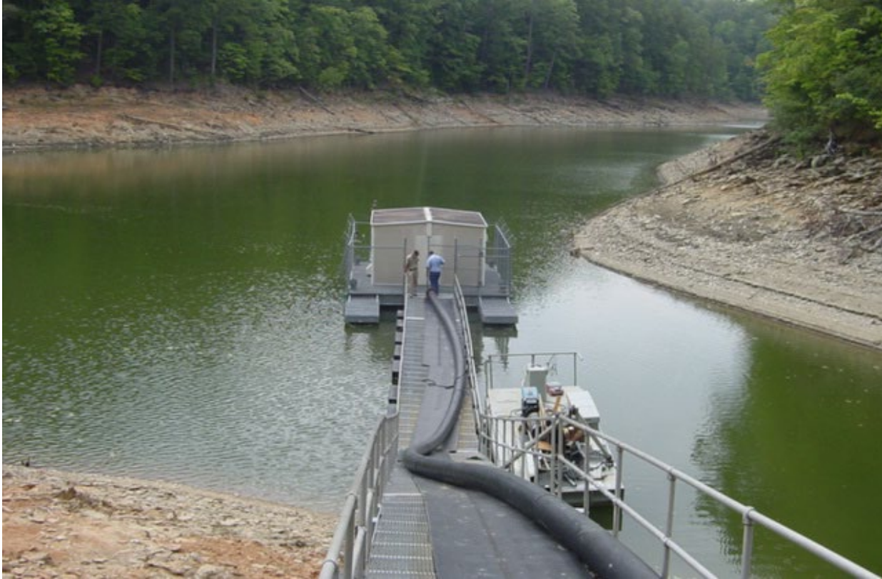
Figure 8-1. The city of Chatsworth Water Intake Structure
