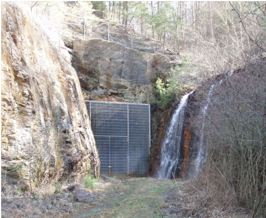
Figure 2-13. Downstream Opening of the Emergency Sluice Tunnel
