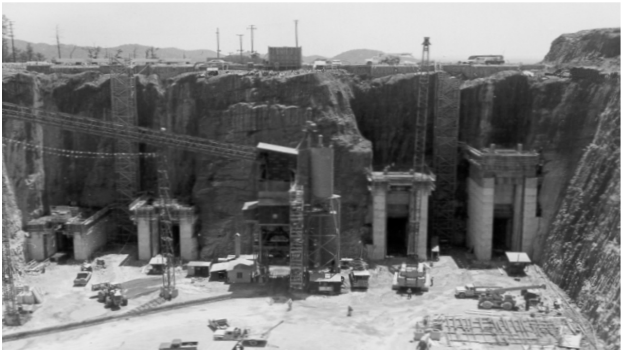
Figure 2-8. Upstream of Intake During Construction, Circa 1974
