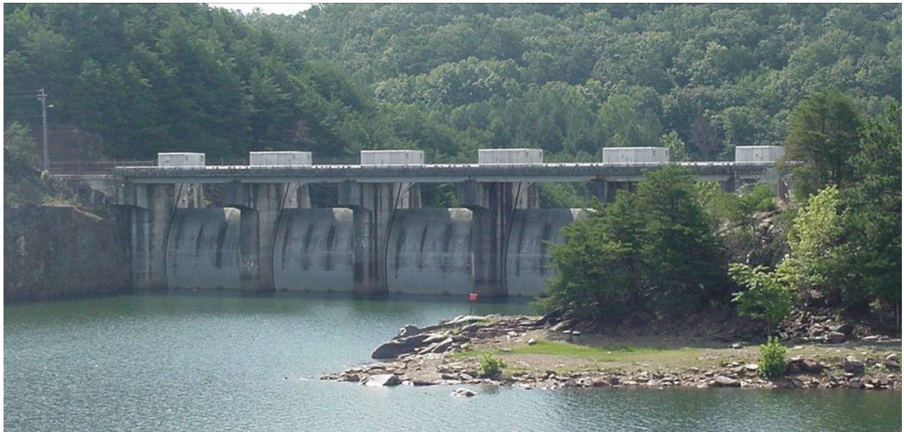
Figure 2-5. Emergency Gated Spillway (Looking Downstream)
