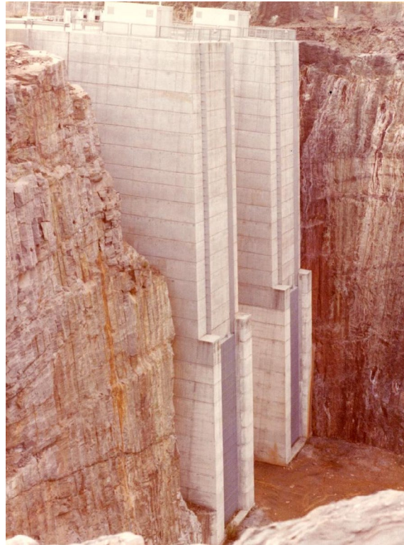
Figure 2-9. Right Bank Intake Prior to Filling, Circa 1974
