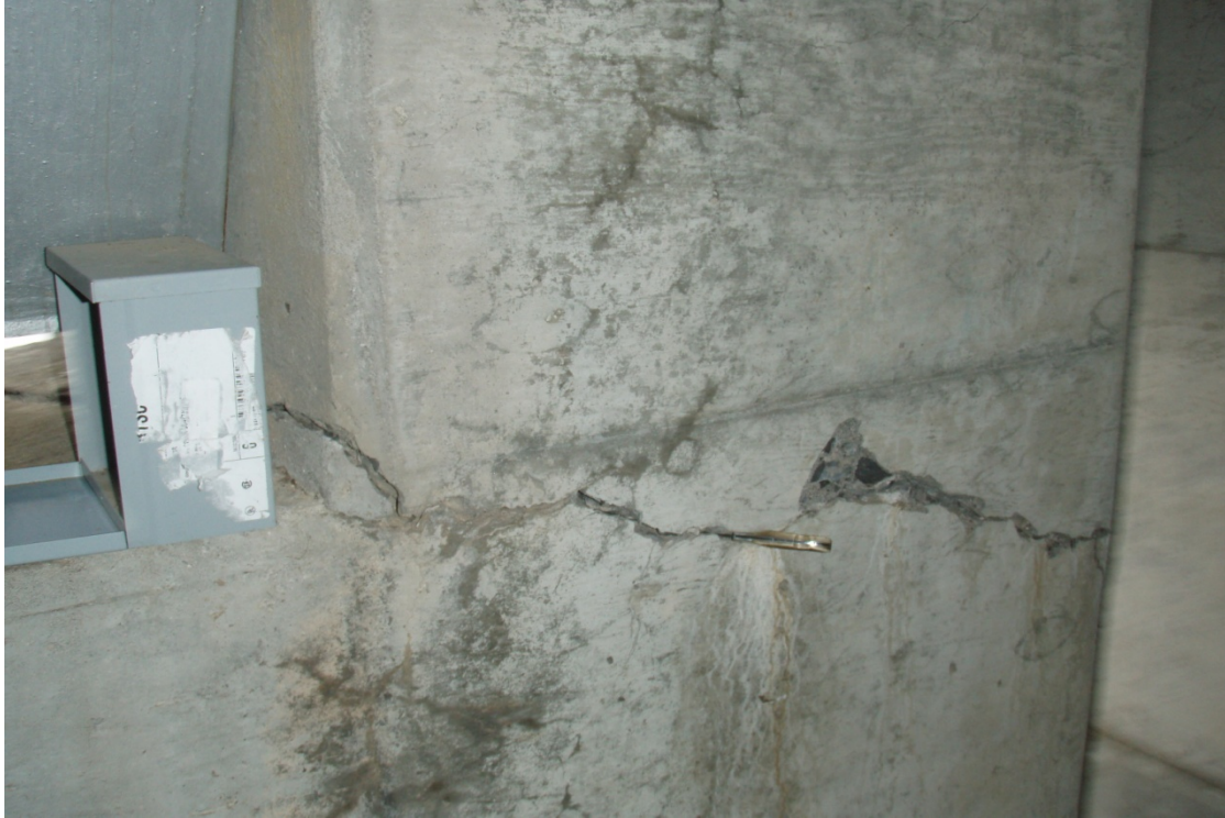
Figure 3-4. Close-up of the Crack on the Upstream Side of Gate No. 4
