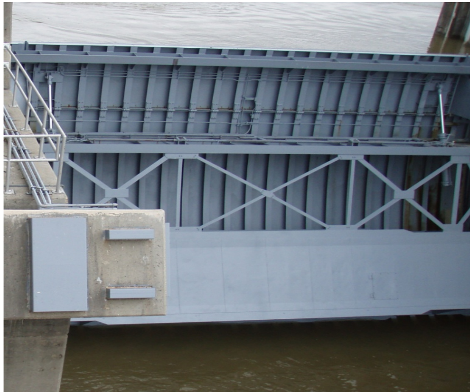
Figure 3-1. Trash Gate at R. F. Henry Dam
