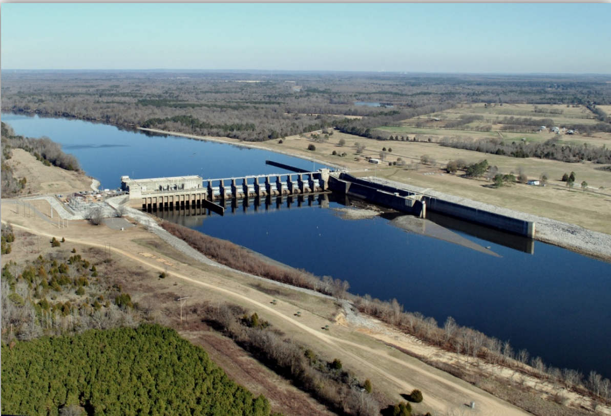
Figure 2-1. R. F. Henry Lock and Dam
