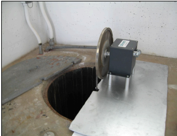
Figure 5-1. Encoder with Wheel Tape for Measuring River Stage or Lake Elevation in the Stilling Well
