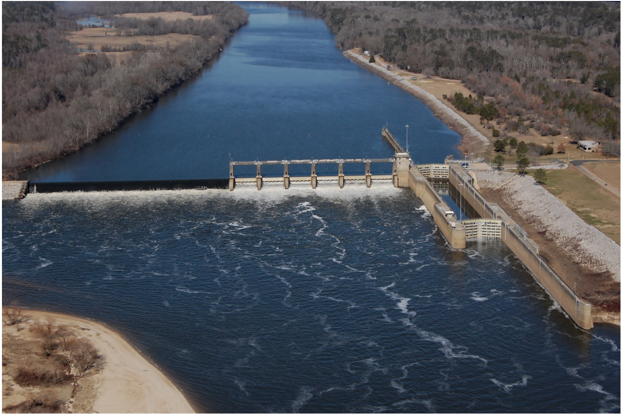
Claiborne Lock and Dam Alabama River, Alabama
