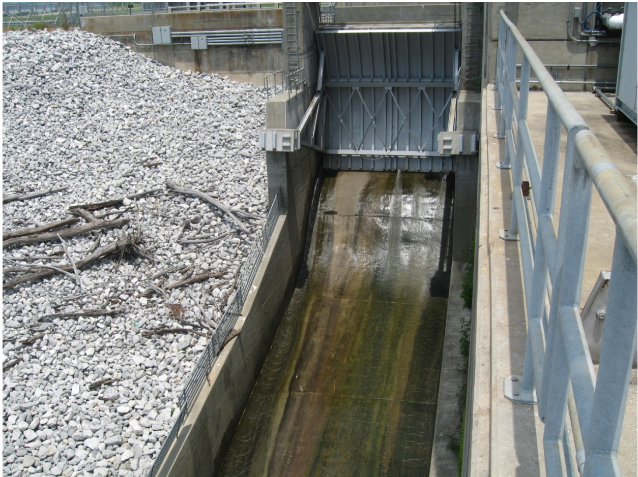
Figure 3-1. Trash Gate at Millers Ferry Project
