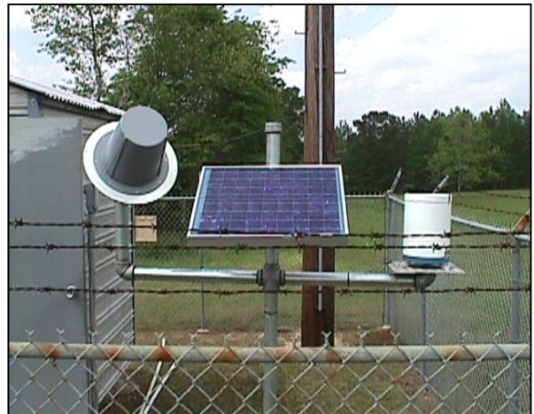
Figure 5-2. Typical Field Installation of a Precipitation Gage
