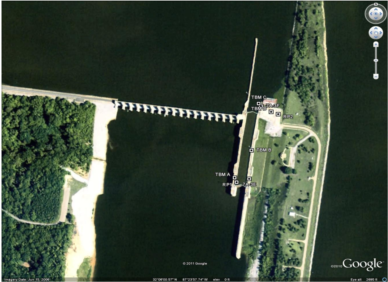
MILLERS FERRY LOCK AND DAM
