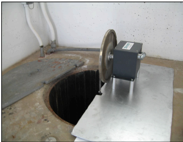
Figure 5-1. Typical Encoder with Wheel Tape for Measuring the River Stage or Lake Elevation in the Stilling Well
