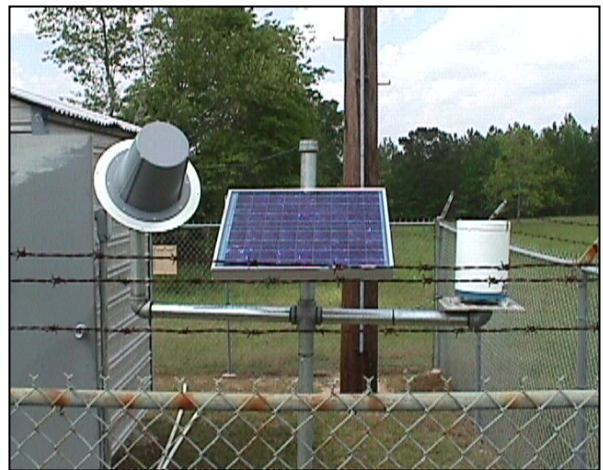
Figure 5-2. Typical Field Installation of a Precipitation Gage
