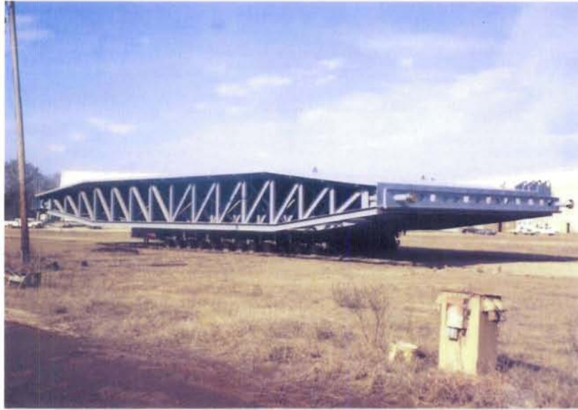
Figure 3 Lock Gate Moving to Barge
