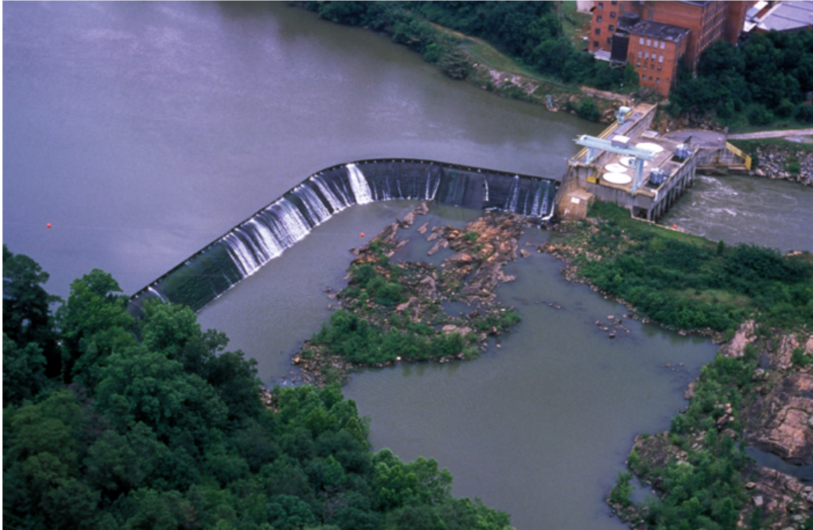
Figure F.29 Photo of North Highlands Dam
