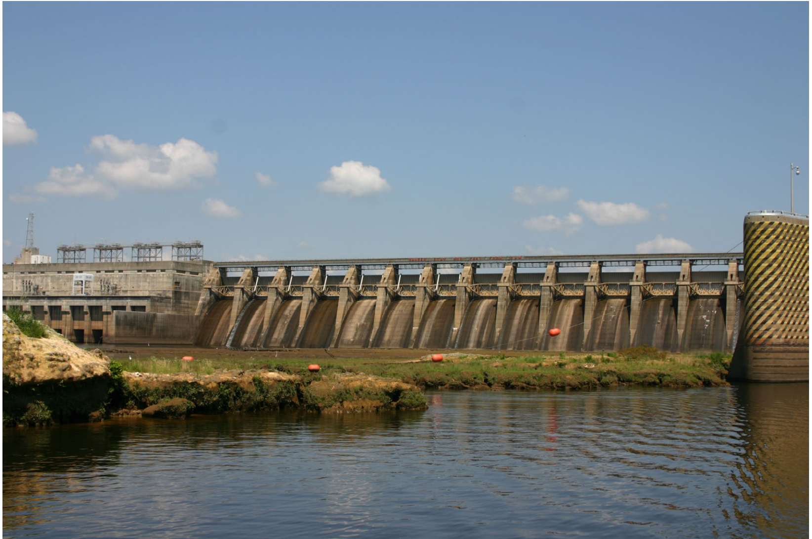
Figure C.02 Photo of Walter F. George Dam
