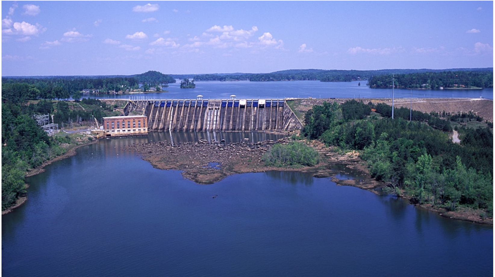
Figure F.09 Photo of Bartletts Ferry Dam
