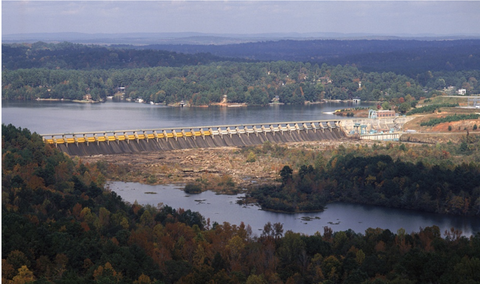
Figure F.23 Photo of Oliver Dam
