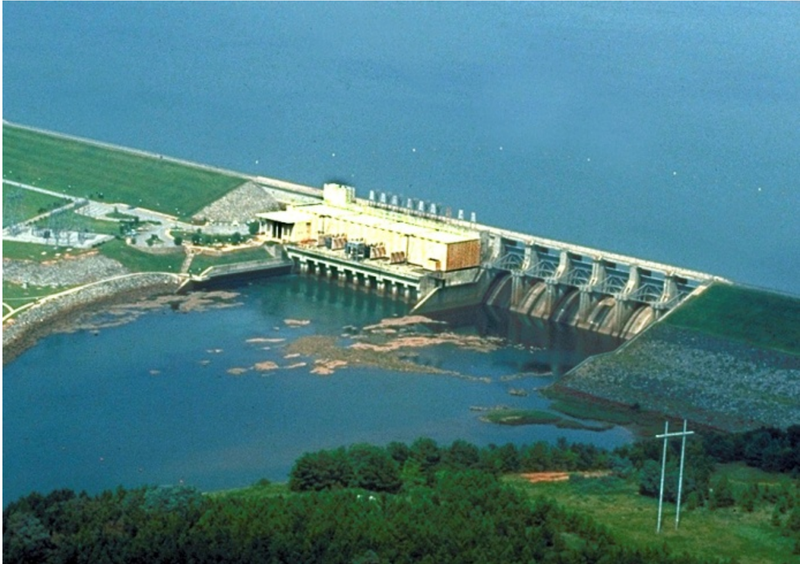
Figure B.02 Photo of West Point Dam
