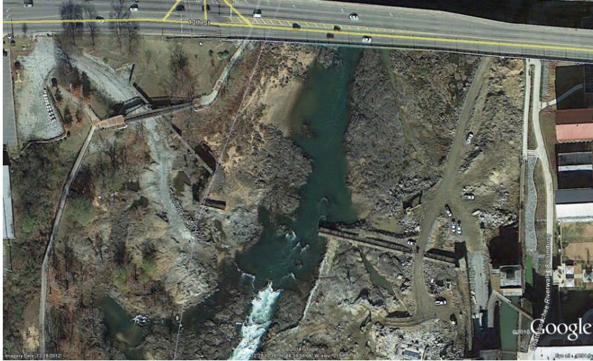
1 2 3 Figure 4-18. Eagle and Phenix Dam after Breach (Photograph courtesy of Google Earth)
