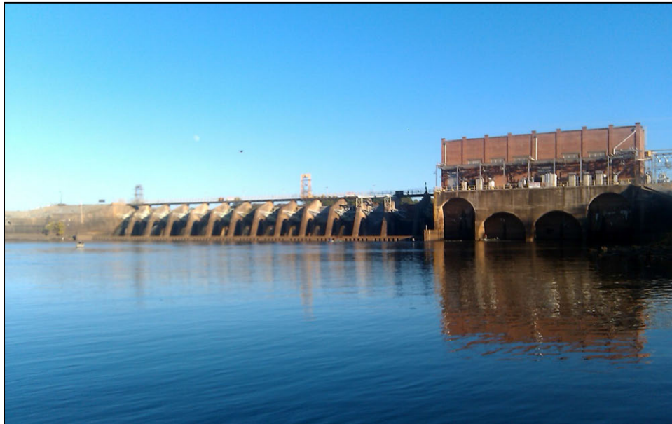
9 10 Figure 4-19. Crisp County Dam
