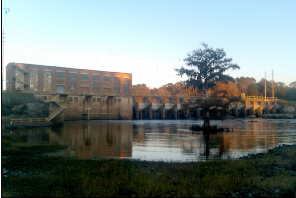
1 2 Figure 4-20. Flint River Dam
