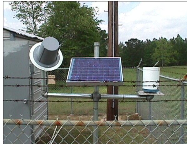
Figure 5-2. Typical Field Installation of a Precipitation Gage
