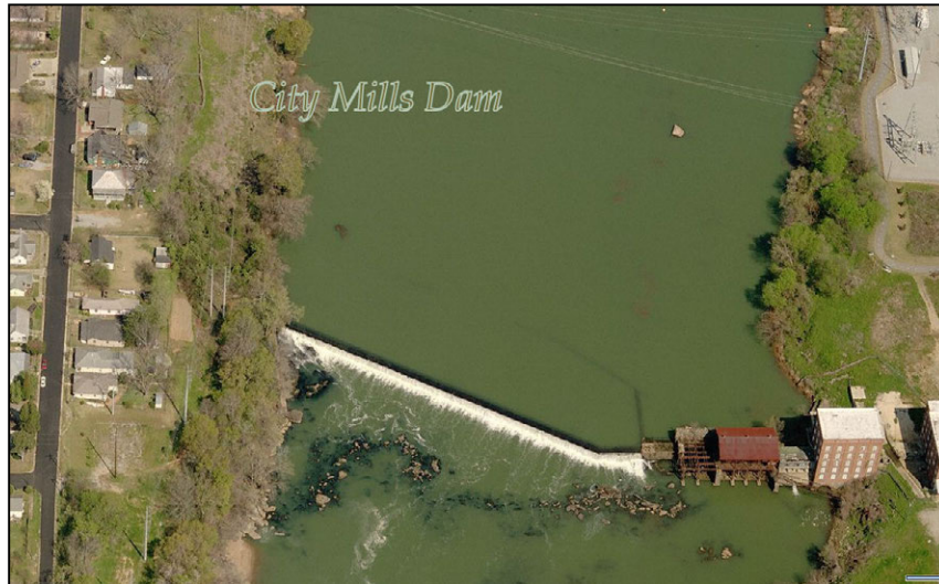
5 Figure 4-16. City Mills Dam (Photograph courtesy of GPC)
