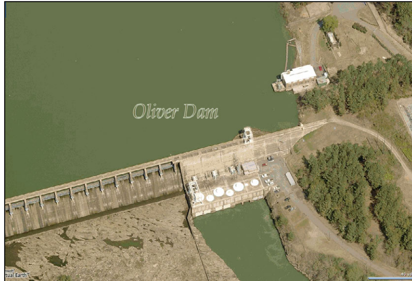
1 2 Figure 4-14. Oliver Dam (Photograph courtesy of GPC)
