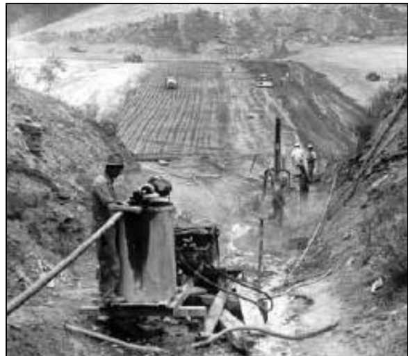
Figure 3-1. Foundation work at Buford Dam (Circa 1950-51)
