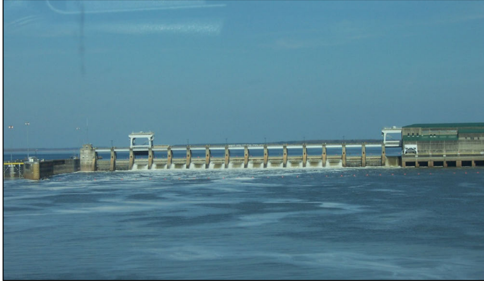
1 2 Figure 4-6. Jim Woodruff Lock and Dam
