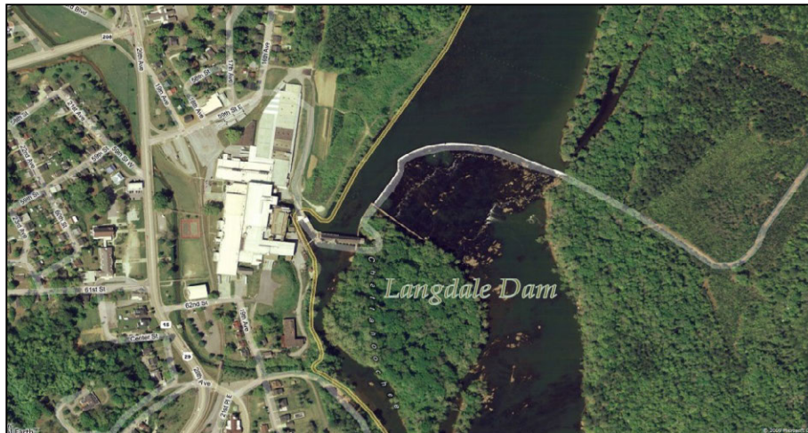
8 9 10 11 12 13 14 15 16 Figure 4-9. Langdale Dam (Photograph courtesy of Google Earth)
