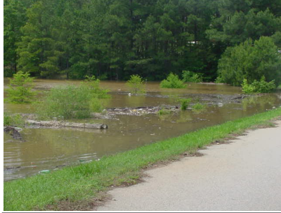
Holiday Campground Causeway at 639.46 feet NGVD29
