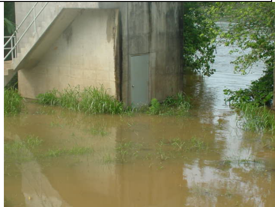
West Point water intake structure. Photo taken at 36,650 cfs.
