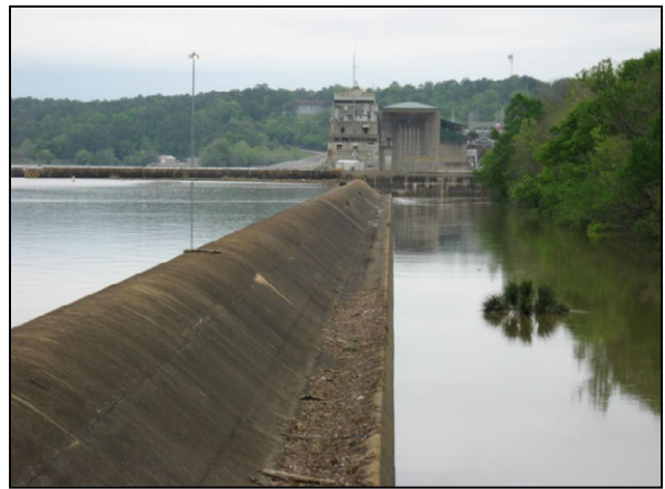
Figure 2-3. Fixed-Crest Spillway without Flow Over the Top
