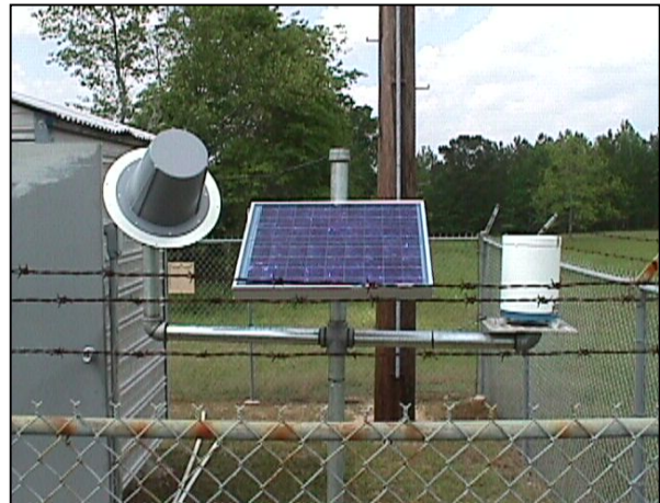
Figure 5-2. Typical Field Installation of a Precipitation Gage
