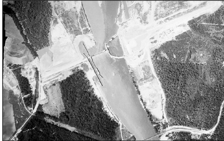
Figure 3-1. Cofferd Dam Protecting the Powerhouse Construction, Circa 1952-53
