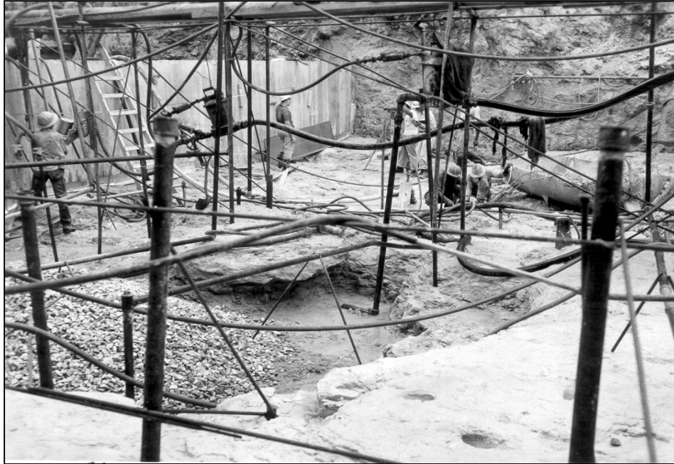
Figure 3-7. Well points for dewatering the work area, Circa 1955-56
