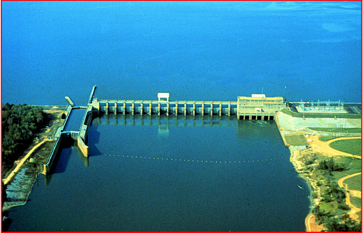
Jim Woodruff Lock and Dam
