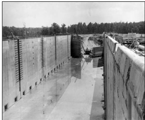
Figure 2-6. Lock Under Construction, Circa 1952-53
