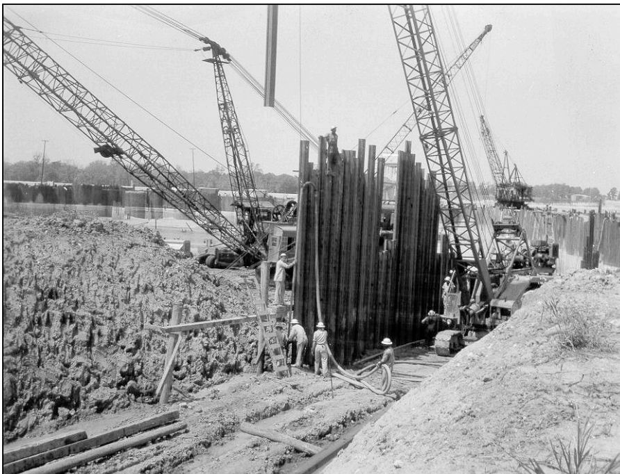
Figure 3-4. Sheet Piling Being Driven in Place, Circa 1955-56
