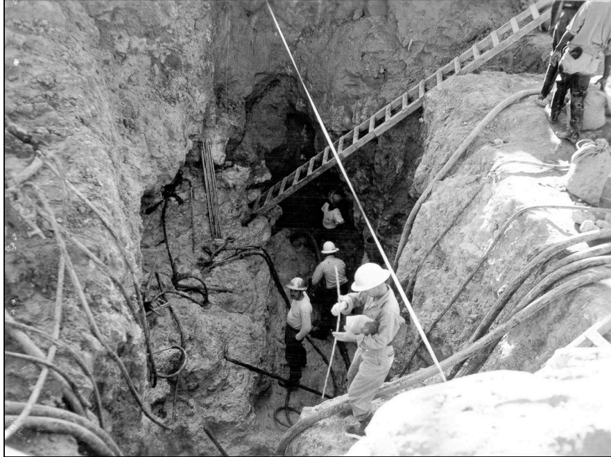
Figure 3-5. Joint Cavity Under the Foundation Area, Circa 1955-56
