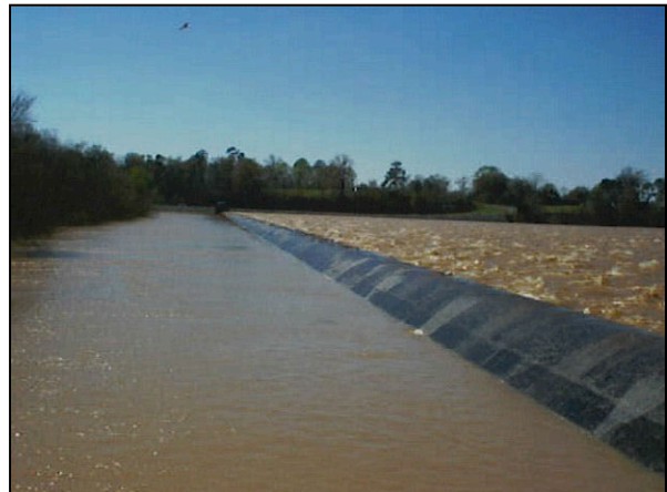
Figure 2-4. Fixed-Crest Spillway with Waves Splashing Over the Top
