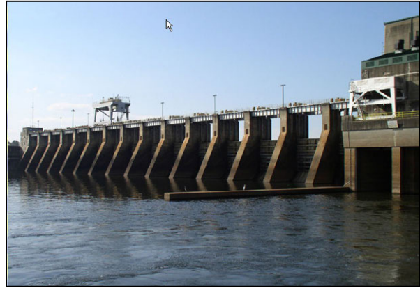
Figure 2-2. Jim Woodruff Spillway Gates
