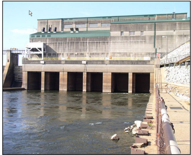
Figure 2-5. Powerhouse and Tailrace
