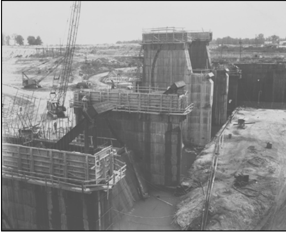
Figure 3-2. Gate Supports, Circa 1961-62
