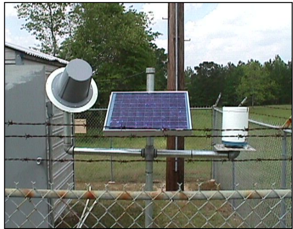
Figure 5-2. Typical Field Installation of a Precipitation Gage
