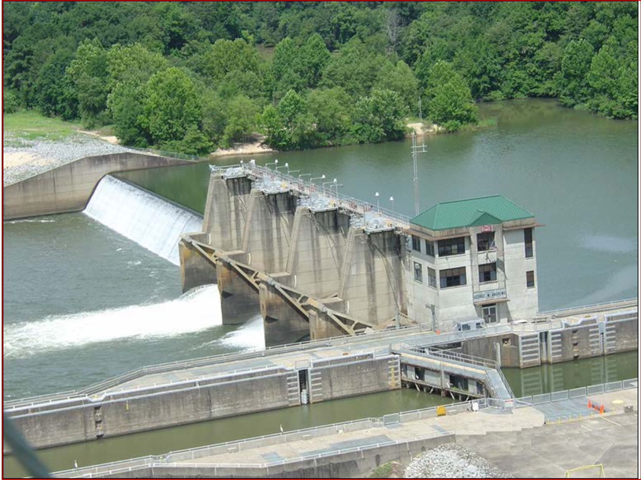
George W. Andrews Lock and Dam
