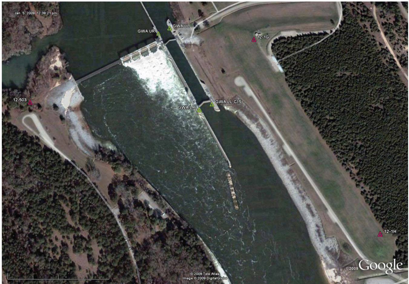
George W. Andrews Lock and Dam
