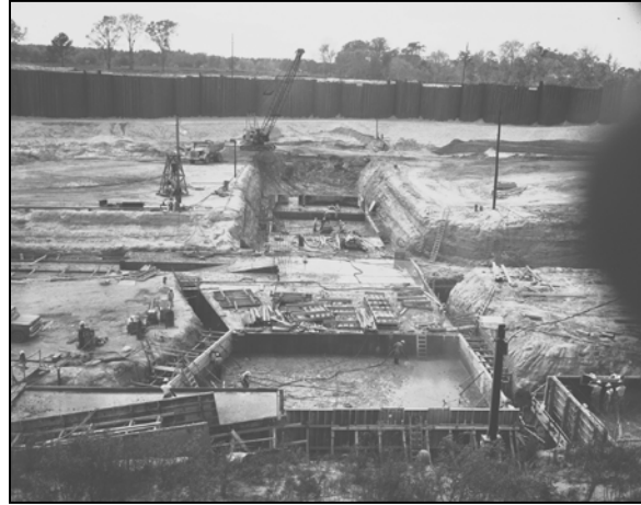
Figure 3-3. Foundation for Miter Gate, Circa 1961-62
