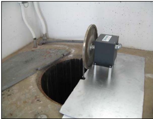
Figure 5-1. Encoder with Wheel Tape for Measuring the River Stage or Lake Elevation in the Stilling Well
