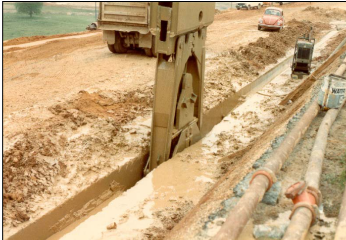
Figure 3-6. Trench Excavation for Cutoff Wall
