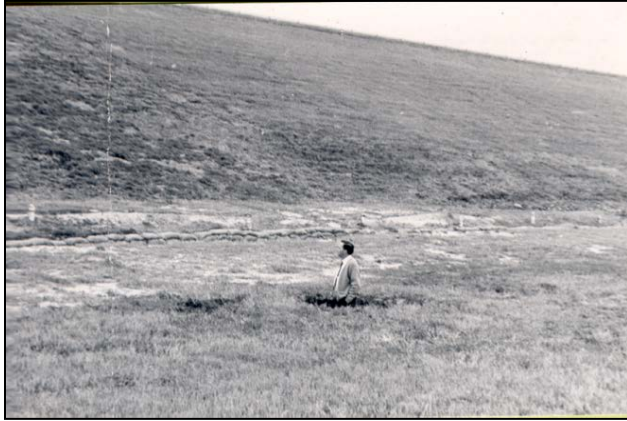
Figure 3-1. Man Standing in Sinkhole
