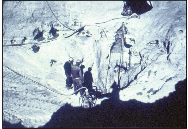
Figure 3-2. Cavern in Foundation Area
