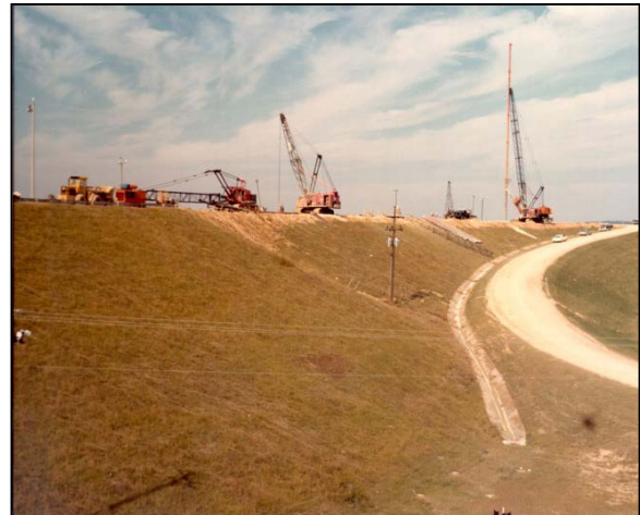
Figure 2-3. Earth dikes during construction of cutoff wall
