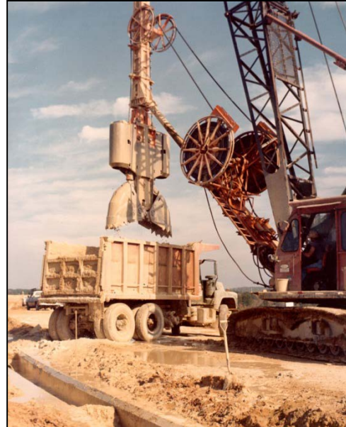
Figure 3-7. Cutoff Wall Construction
