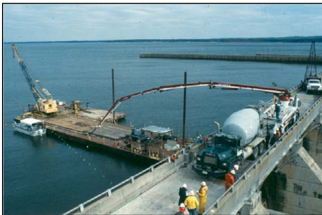
Figure 3-5. Boom Supplying Grouting Operation
