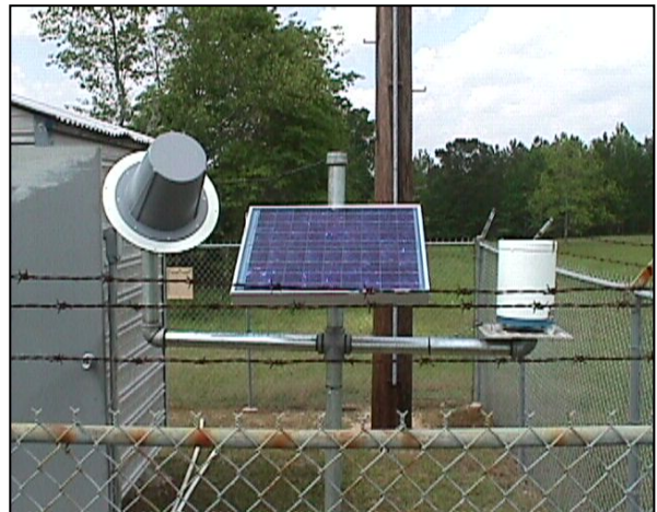
Figure 5-2. Typical Field Installation of a Precipitation Gage
