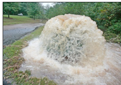
Storm drain overflow, Roswell, GA
