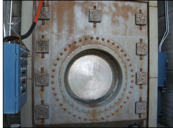
Figure 2-6. Broome-type Sluice Gate
