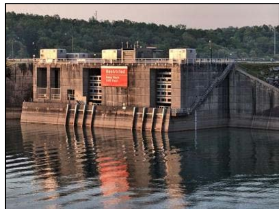
Figure 2-5. Intake Structure
