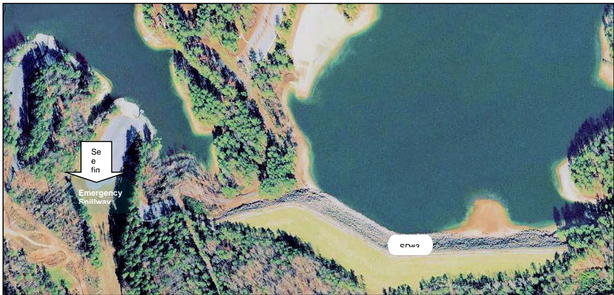
Figure 2-3. Saddle Dike No. 3 and Emergency Spillway
