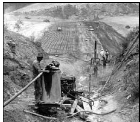
Figure 3-6. Main Dam Construction, 1952
