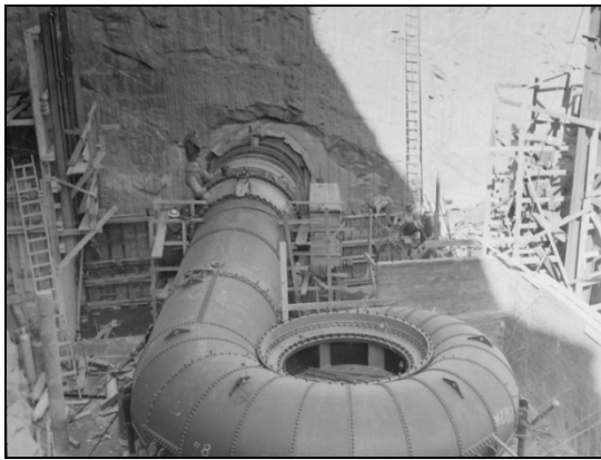
Figure 3-4. Steel Penstock and Scroll Case, 1953
