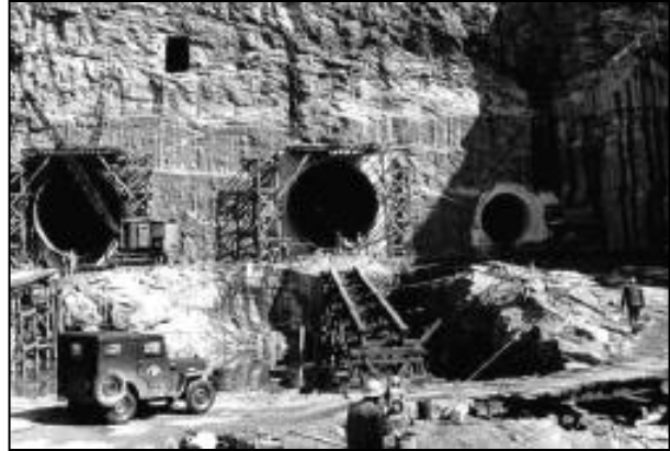
Figure 3-3. Penstock Construction, 1953
