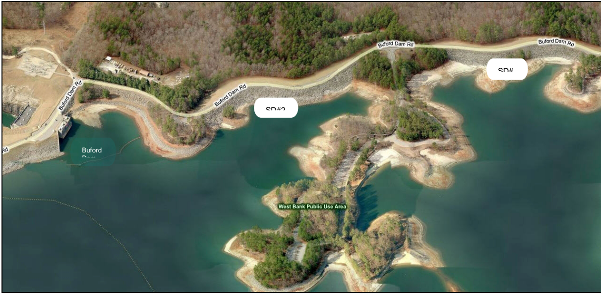
Figure 2-2. Saddle Dikes No. 1 and No. 2.
