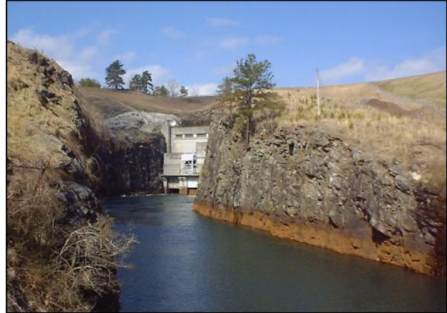
Figure 2-7. Powerhouse and Discharge Channel
