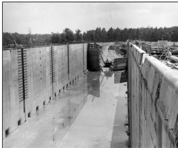
Figure 2-6. Lock Under Construction, Circa 1952-53
