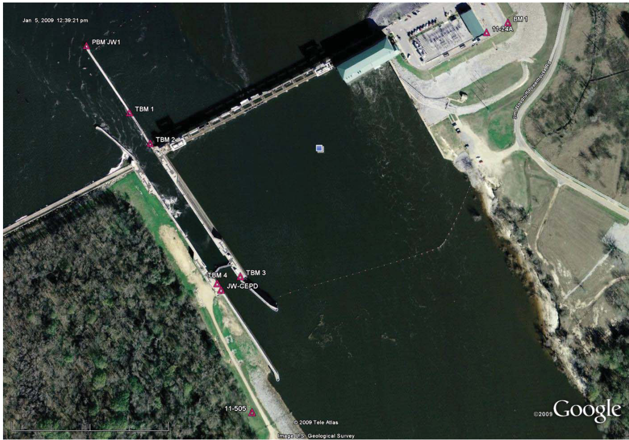
Jim Woodruff Lock and Dam
