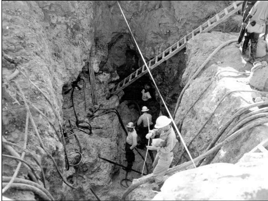
Figure 3-5. Joint Cavity under the Foundation Area, Circa 1955-56
