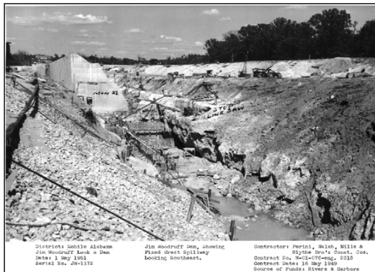
Figure 3-2. Construction of the Monolith, Circa May 1951
