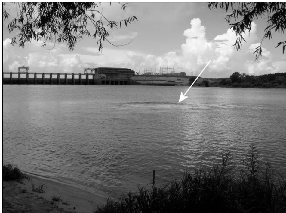
Figure 3-8. Boil in the River Caused by Underground Flow from the Reservoir
