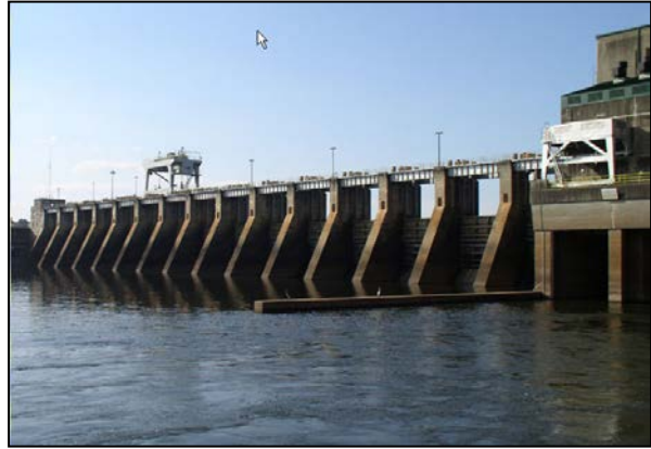
Figure 2-2. Jim Woodruff Spillway Gates
