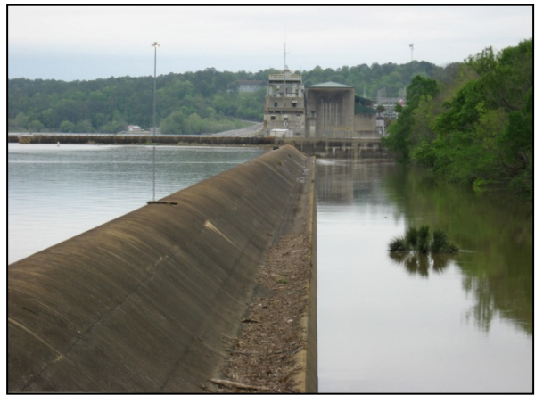
Figure 2-3. Fixed-Crest Spillway without Flow Over the Top
