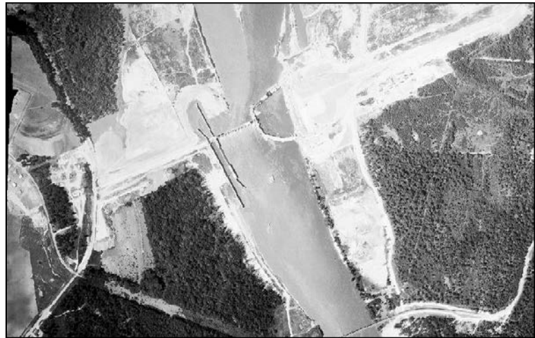
Figure 3-1. Cofferd Dam Protecting the Powerhouse Construction, Circa 1952-53
