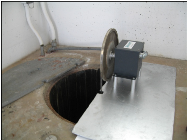
Figure 5-1. Encoder with Wheel Tape for Measuring the River Stage or Lake Elevation in the Stilling Well
