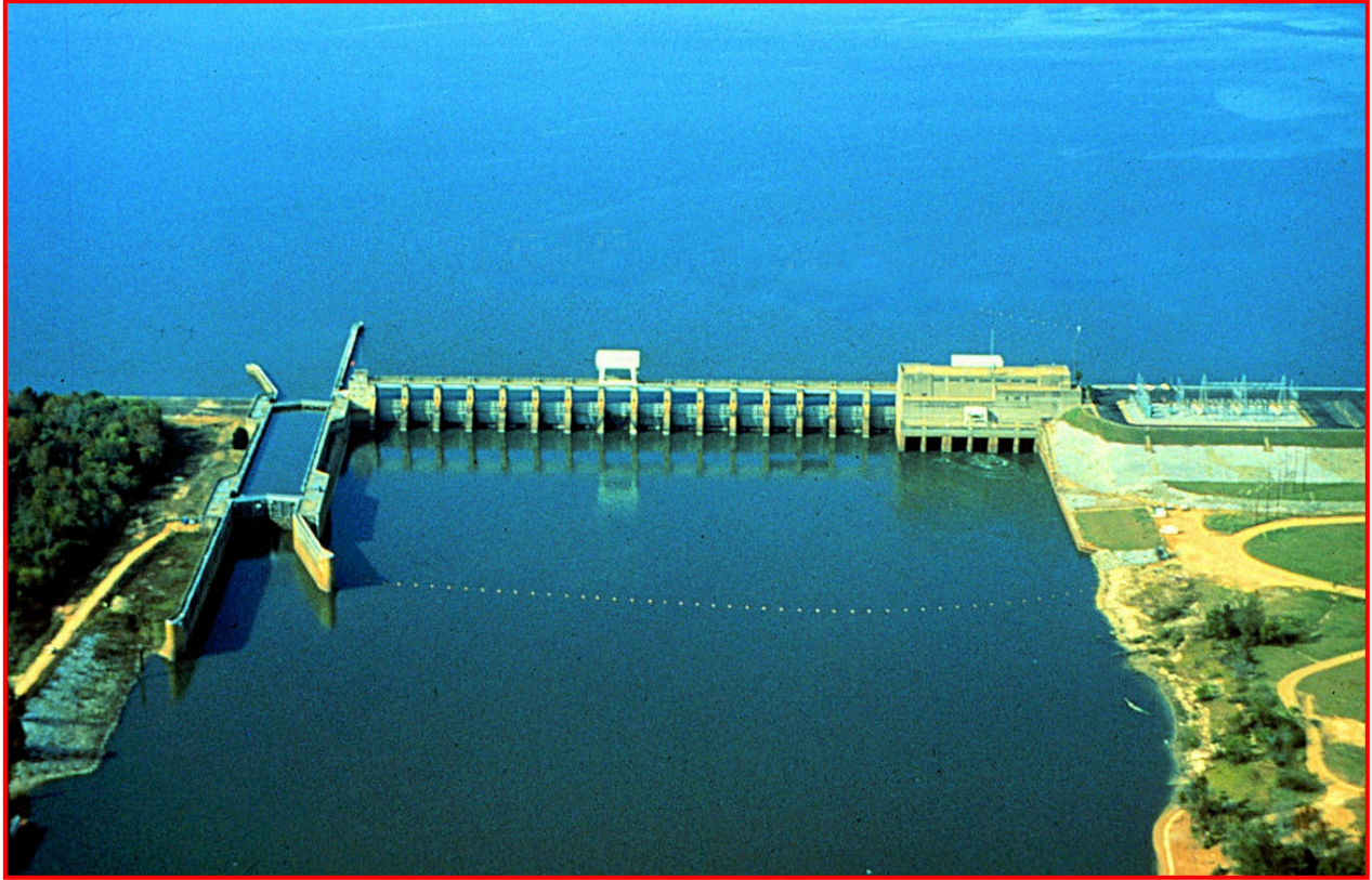
Jim Woodruff Lock and Dam
