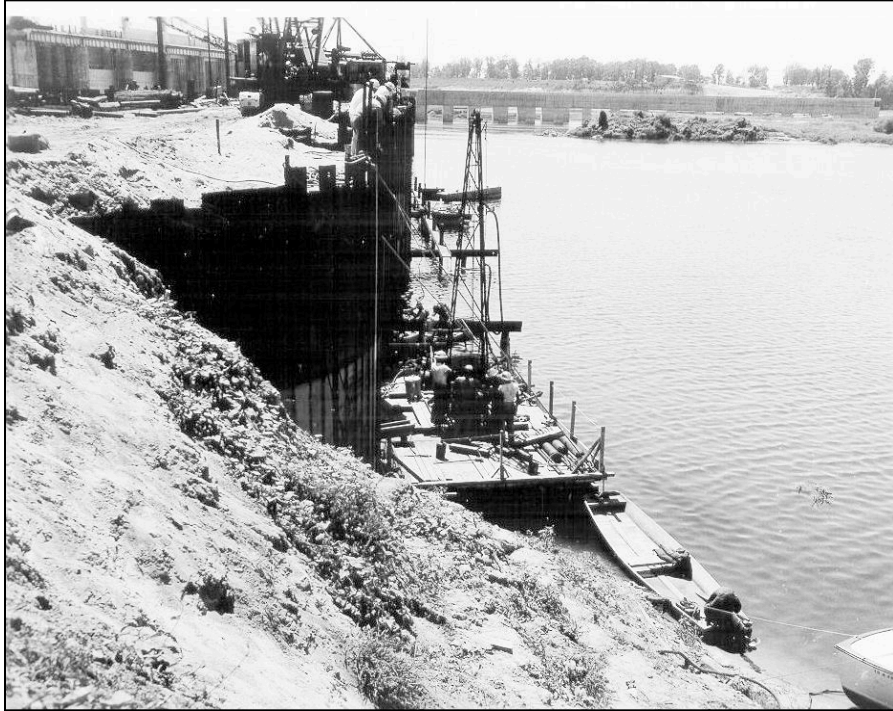
Figure 3-3. Sheet Piling Upstream of the Powerhouse and Grouting Crew Pouring Grout into the Cavern, Circa 1955-56
