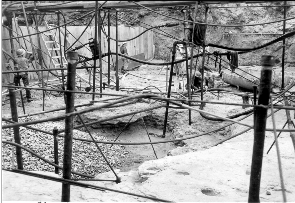
Figure 3-7. Well points for dewatering the work area, Circa 1955-56
