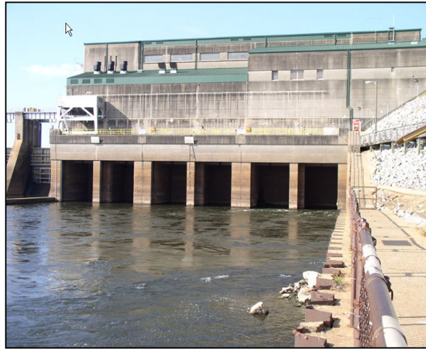
Figure 2-5. Powerhouse and Tailrace
