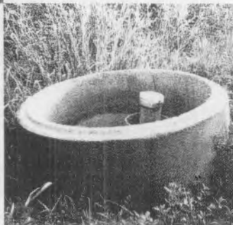
A monitoring well is used to test groundwater quality, in the vicinity of the Francop site.
