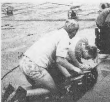
Welded sheets of PEHD plastic are laid as a basic seal to prevent dispersion of contaminants, at the Francop land-based CDF in Hamburg, Germany.
