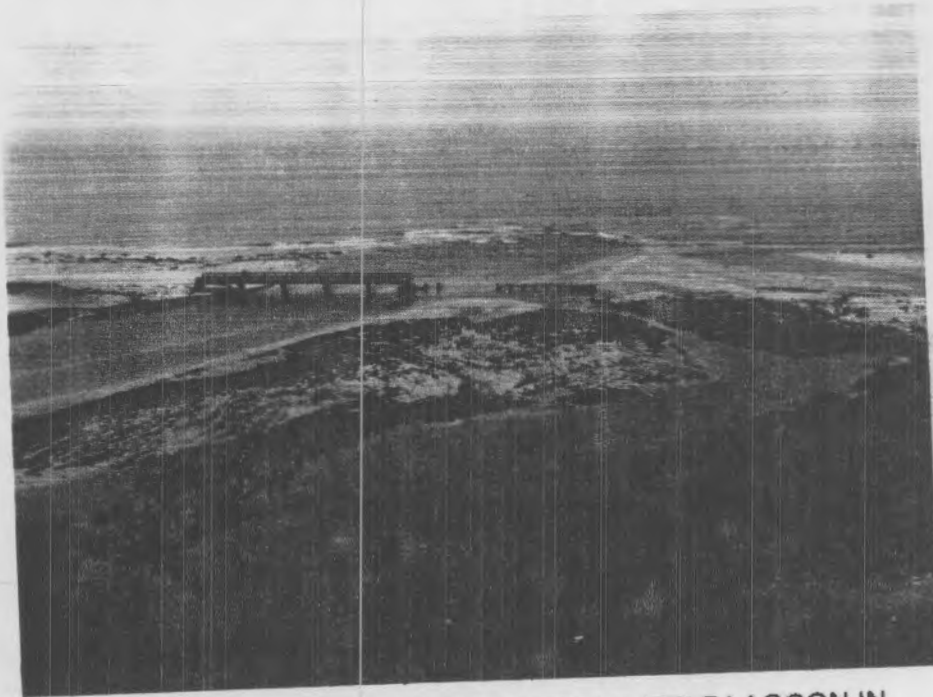
HIGHWAY BRIDGE CROSSING INLET AT LITTLE LAGOON IN BALDWIN COUNTY, ALA. - SEVERAL SPANS COMPLETELY DESTROYED AND ROAD AND BRIDGE APPROACHES WASHED AWAY.
