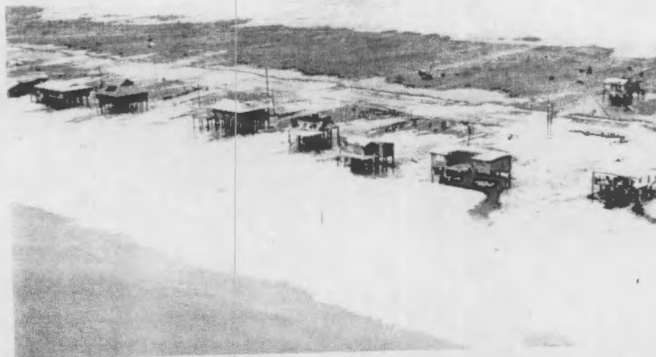
DAUPHIN ISLAND, ALA. LOOKING NORTHWEST. MANY HOMES RECEIVED WIND AND WATER DAMAGE.
