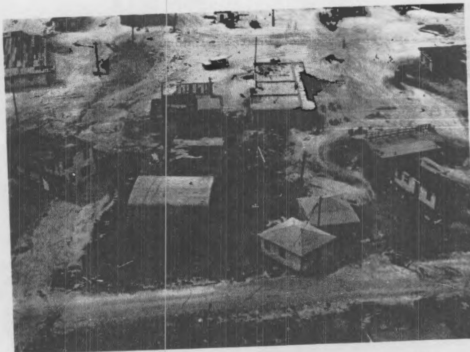
VIEW OF GULF SHORES, ALA. WATER DAMAGE TO HOMES AND BUSINESSES WAS EXTENSIVE. NOTE HOUSE MOVED BY STORM SURGE INTO ROADWAY.
