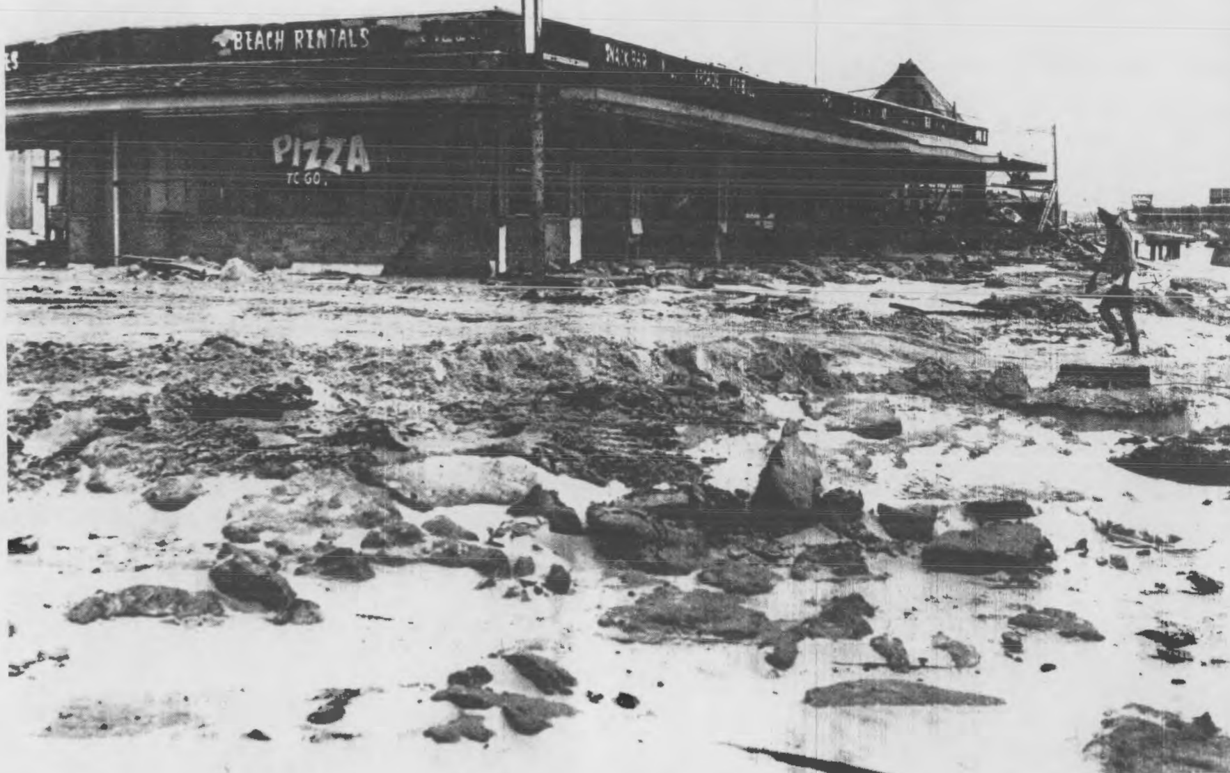
VIEW OF DAMAGE AT THE "HANGOUT," A POPULAR GULF SHORES BEACH ATTRACTION. CHUNKS OF SAND, ASPHALT AND OTHER DEBRIS IN FOREGROUND COVER AN AREA WHICH WAS A SMOOTH PAVED THOROUGHFARE BEFORE HURRICANE FREDERIC.
