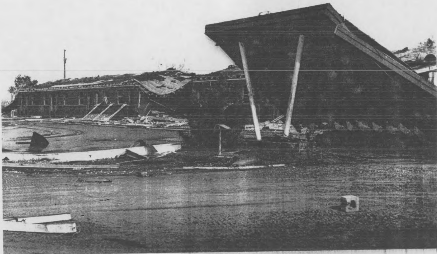
VIEW OF DESTRUCTION AT WOODY'S MOTEL LOCATED ON BATTLESHIP PARKWAY (U.S. HIGHWAY 90 & 98), WHICH CROSSES MOBILE RIVER DELTA IN BALDWIN COUNTY, ALA.
