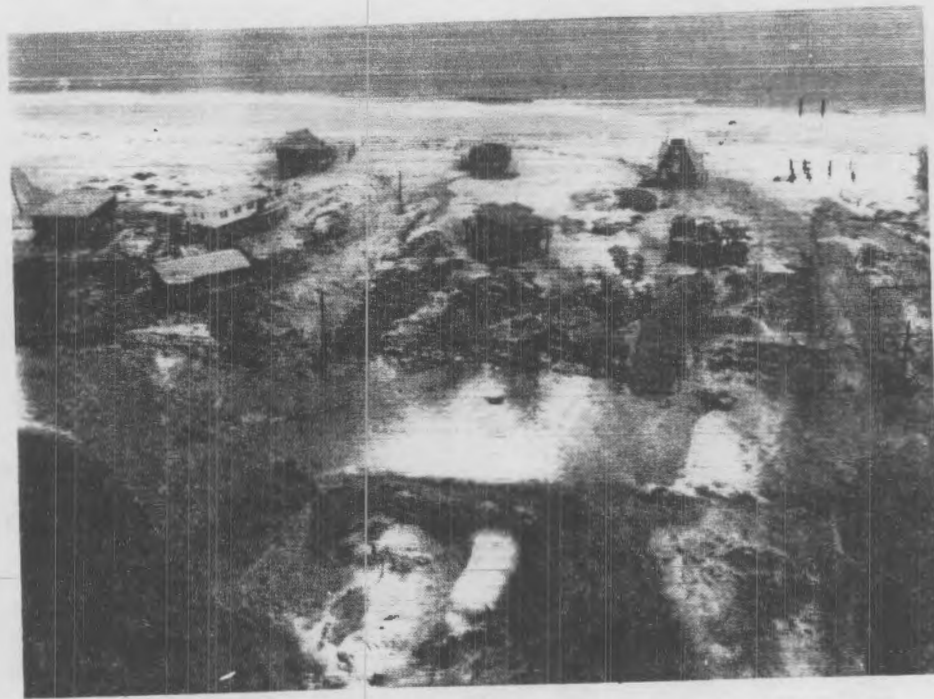
STORM SURGE CAUSED WASHOVER FANS PUSHING SAND ACROSS ROAD INTO MISSISSIPPI SOUND. VIEW OF DAUPHIN ISLAND, ALA. LOOKING SOUTH.
